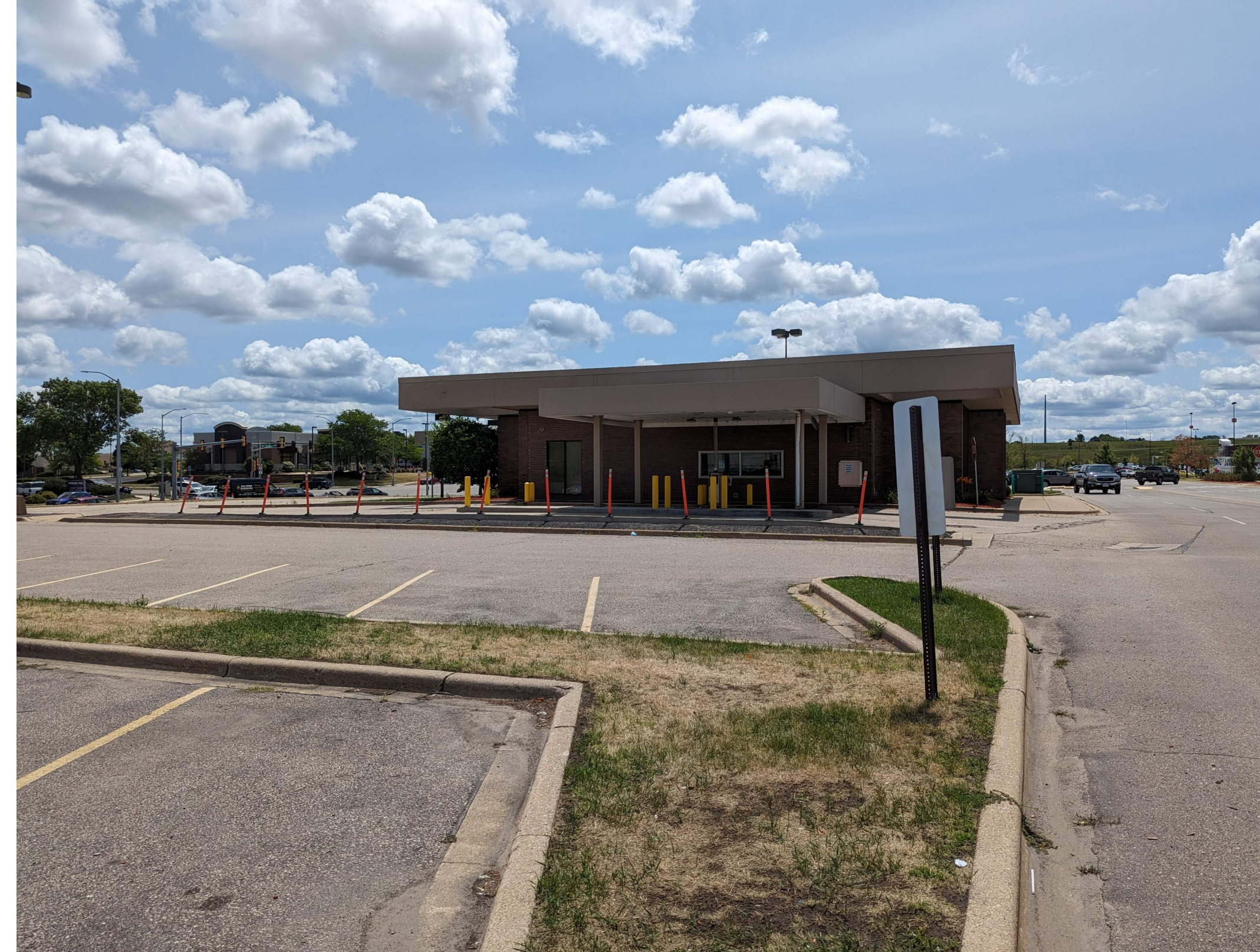
EXISTING NORTH ELEVATION OF CURRENT PROPERTY
