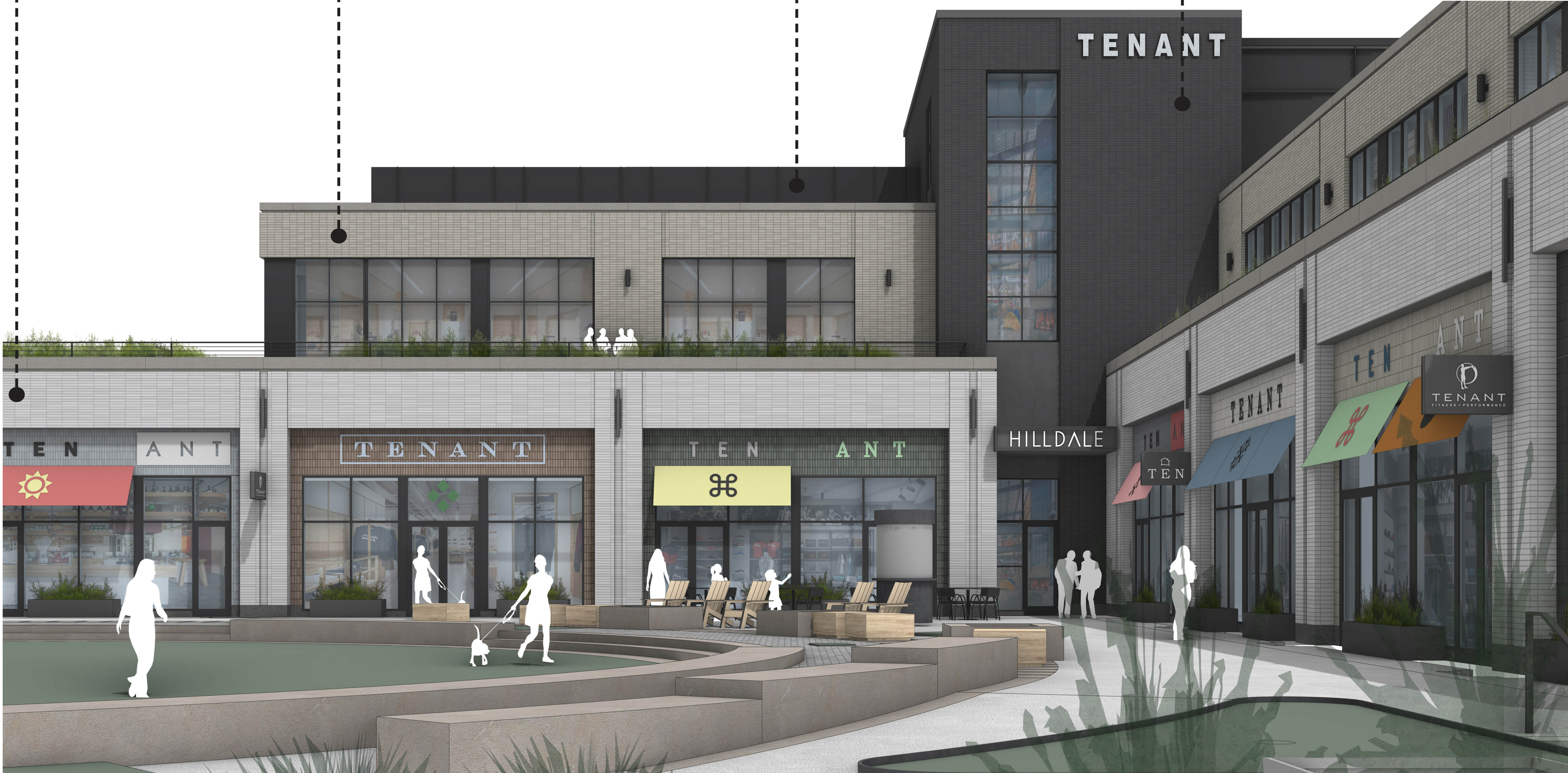
Glen-Gery "Oyster White w/ Speck" 'Saxon' brick (3-5/8" deep, 2-1/4" tall, 15-5/8" wide) comments: 3/8" mortar joint, stacked bond, soldier stacked bond, additional patterns with recessed coursing
