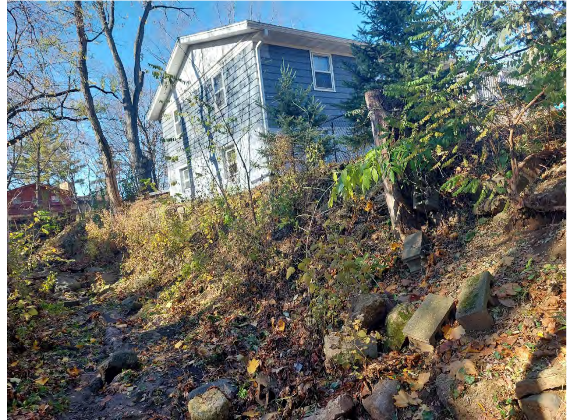
Eroded slope in channel
