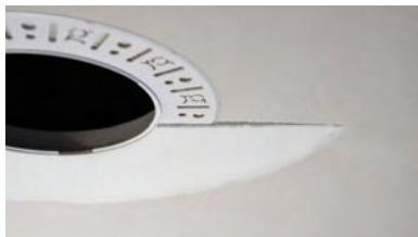
Partially finished mud ring, showing cross-section detail.
