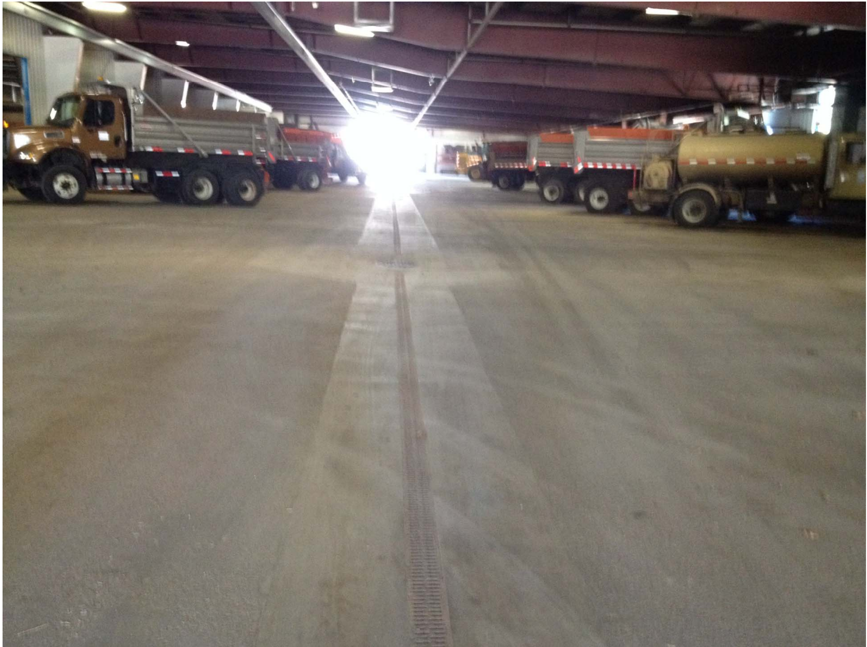
B-1A Indoor vehicle storage – trench drain connected to sanitary sewer
