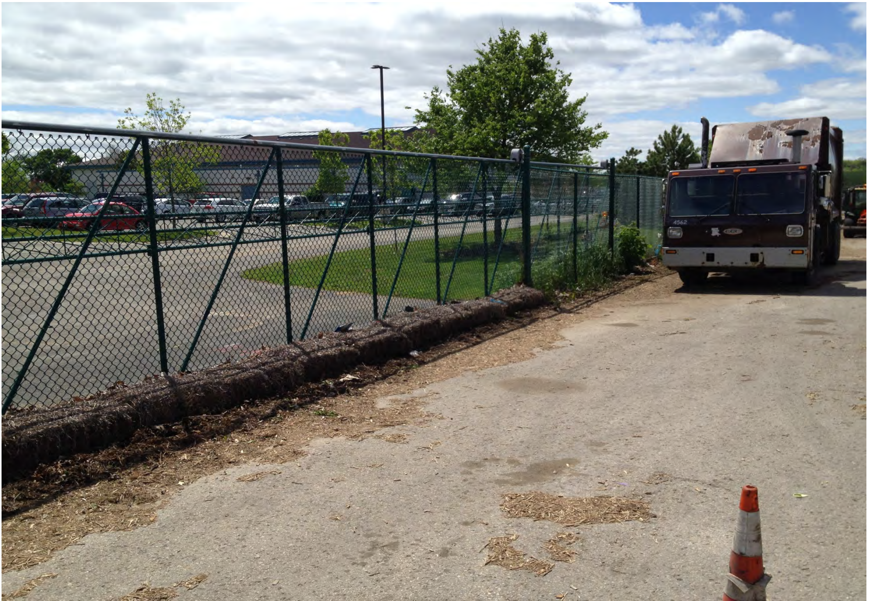
M-2 Vehicle Storage and Parking M-3 Overland flow route with Hay Bales
