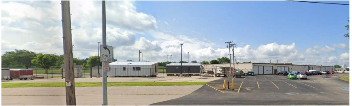
VIEW OF BUILDING B FROM COMMERCIAL AVE
