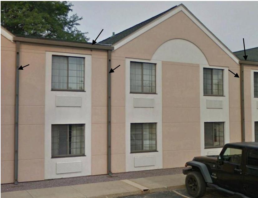
GUTTERS: EPT-2a, TYP DOWNSPOUTS: EPT-1a, TYP
