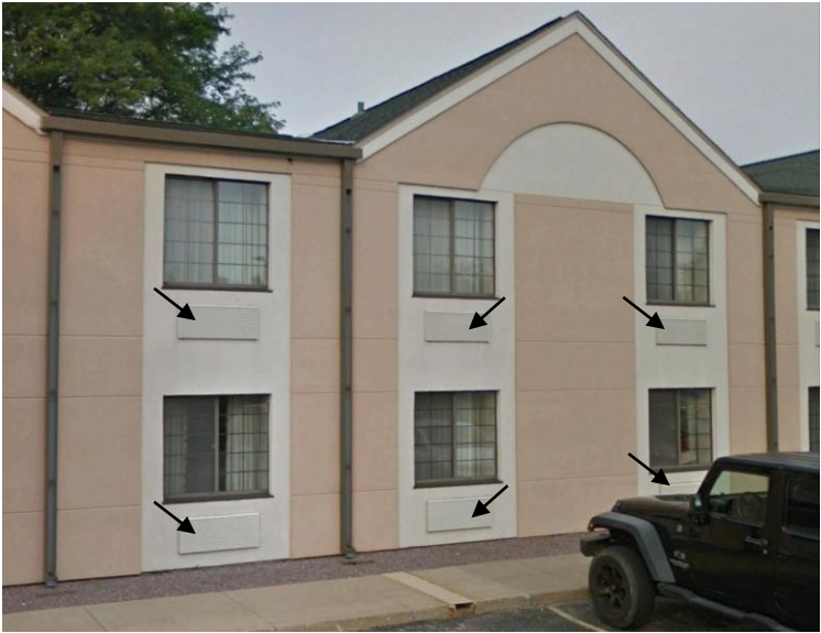
DESCRIPTION: GRILLES FOR PTAC UNIT AIR INTAKE LOCATION(S): UNDER DWELLING UNIT WINDOWS AND SOME OTHER WINDOWS
