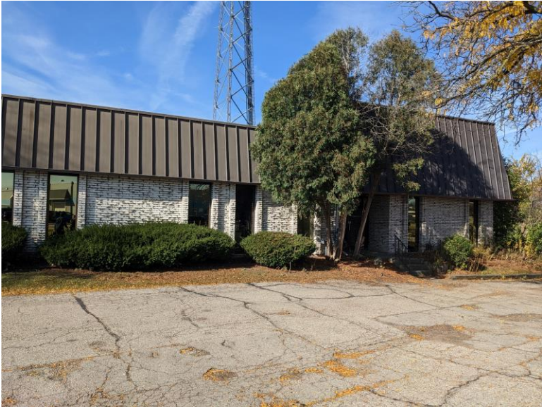
Photo 3: Front of building, parking lot
