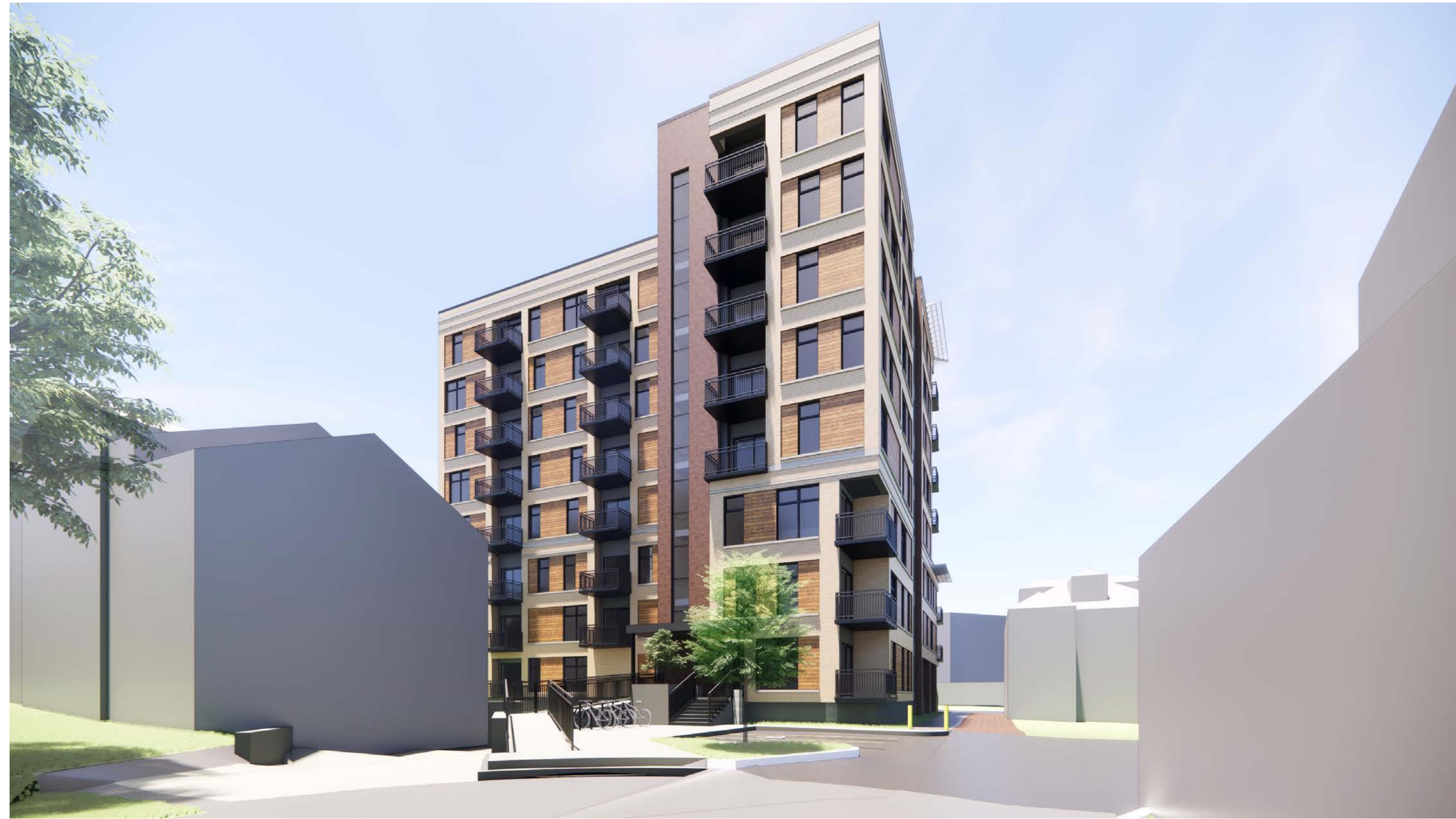
RANDALL CT - LOOKING EAST
