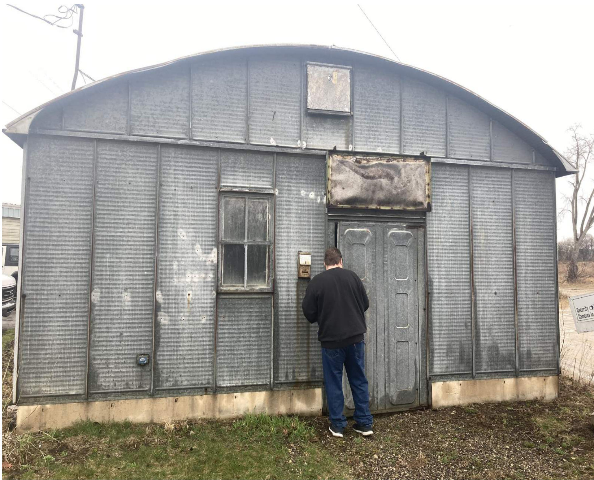
EXISTING METAL SHED
