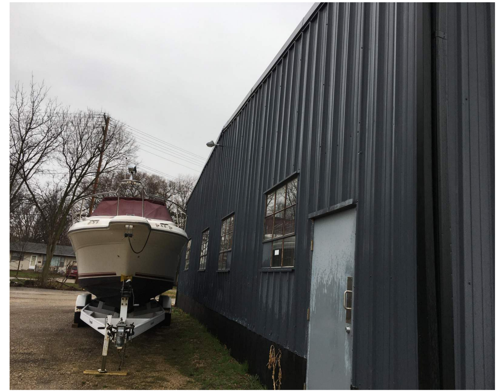
SOUTH SIDE OF EXISTING BUILDING
