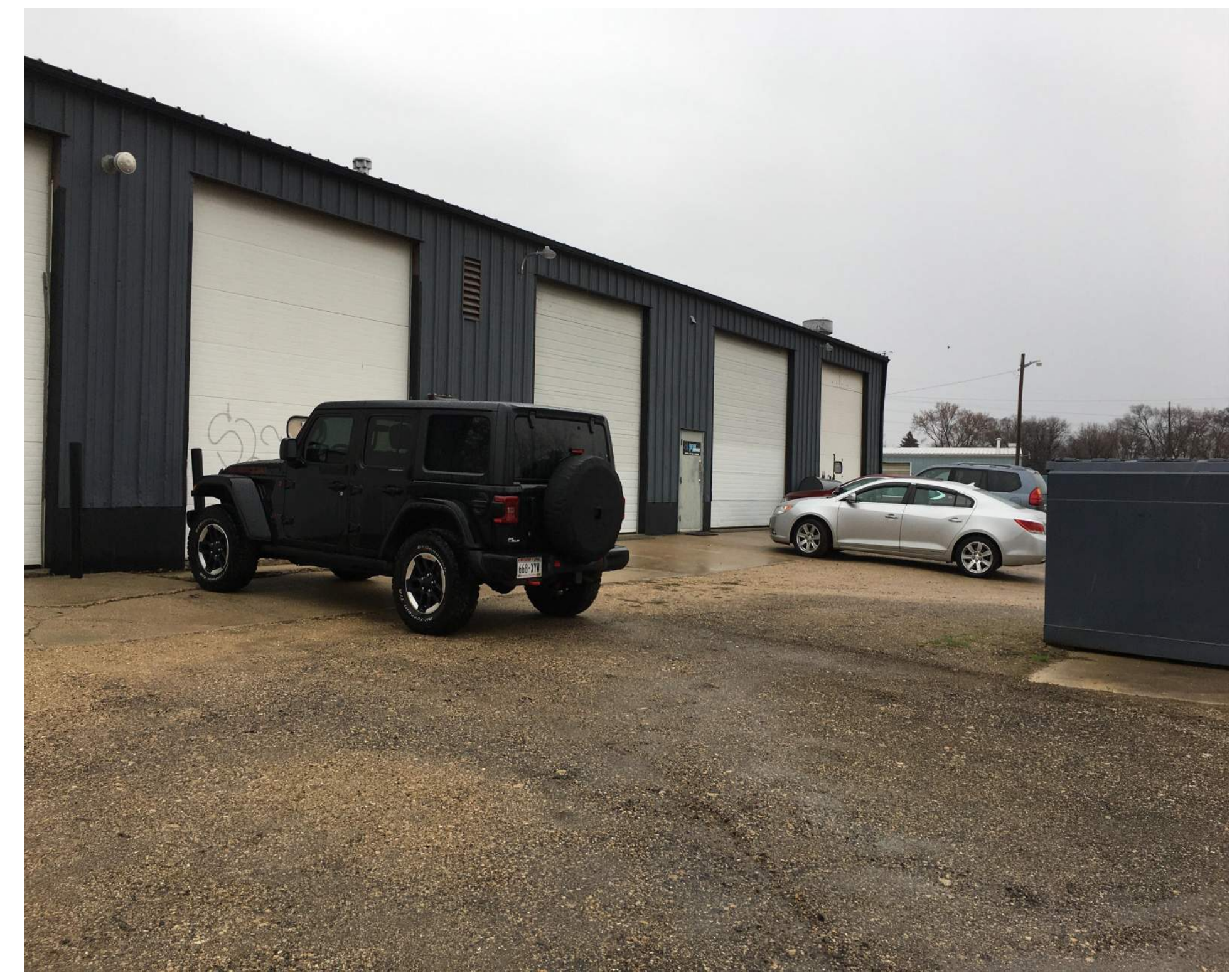
EAST SIDE OF EXISTING BUILDING
