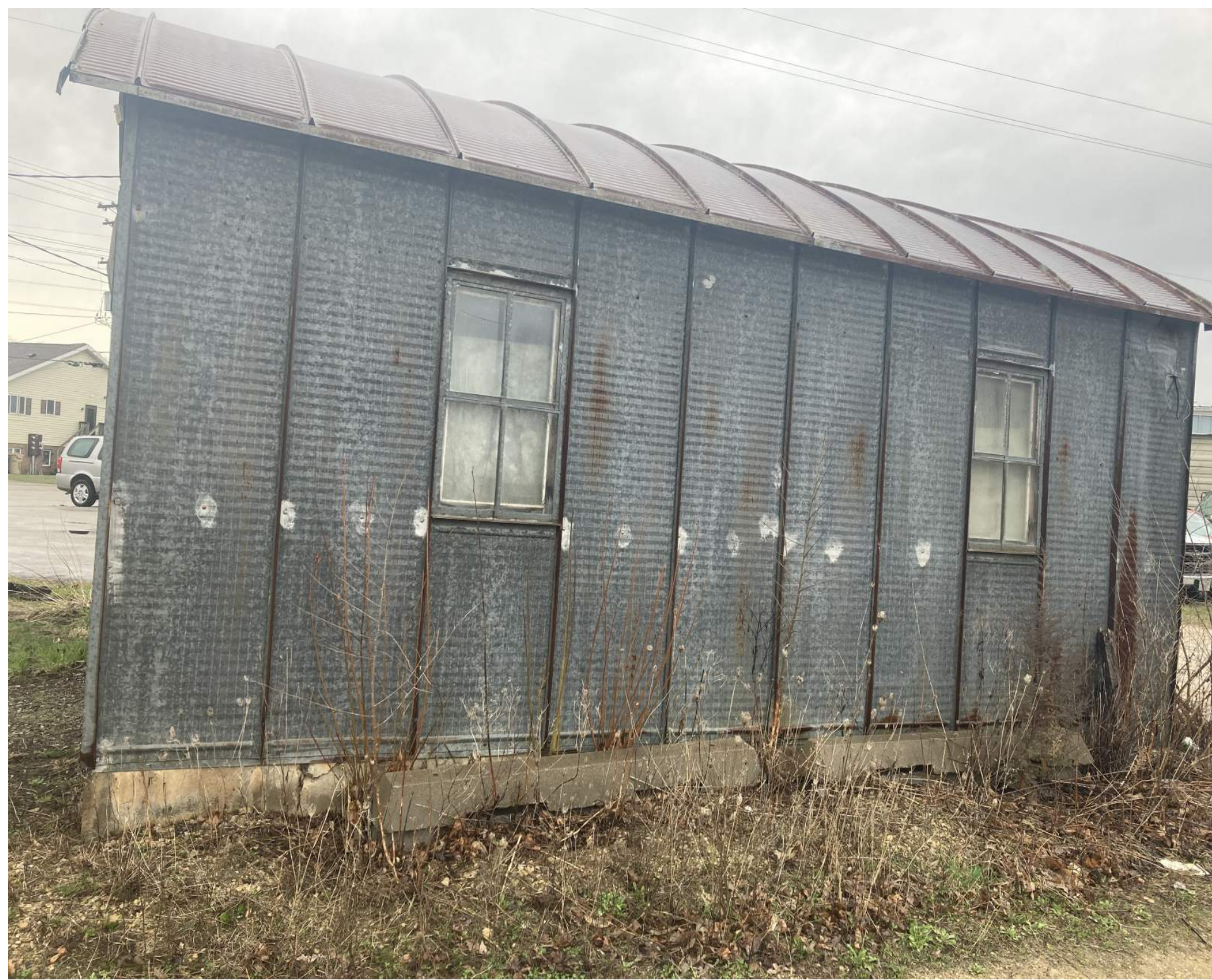
EXISTING METAL SHED
