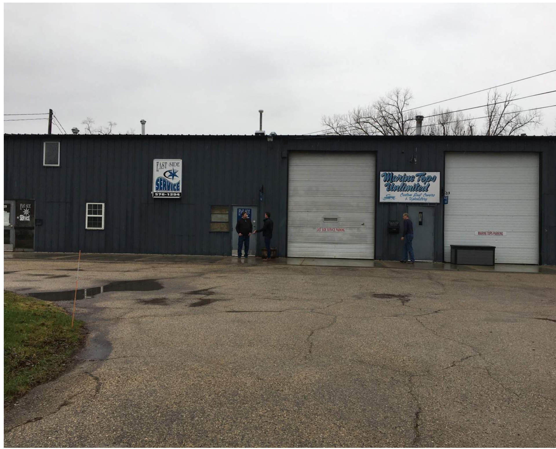
WEST SIDE OF EXISTING BUILDING
