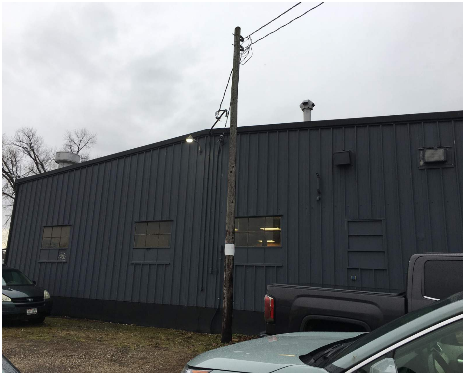
NORTH SIDE OF EXISTING BUILDING
