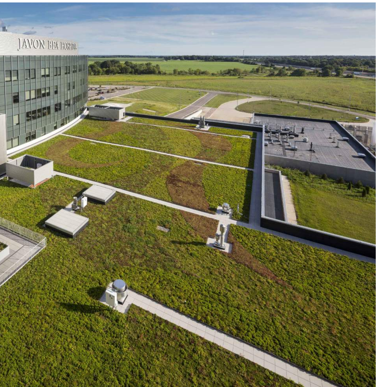
Typical rooftop / penthouse green roof with 2' clear zone around outside edges and mechanical units. Includes additional paver walkways for maintenance access.
