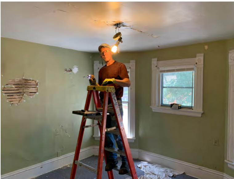
View of Interior Living Space
