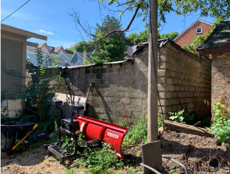
View of back of garage at rear yard
