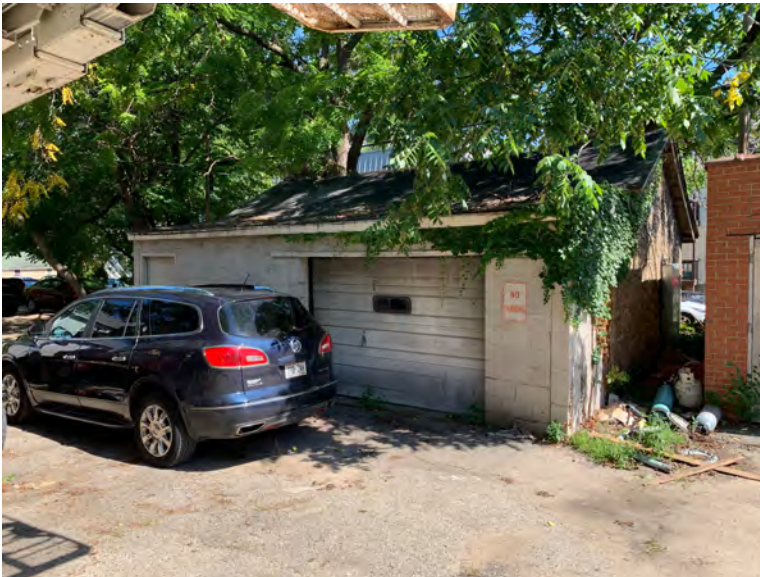
View of detached garage at rear yard
