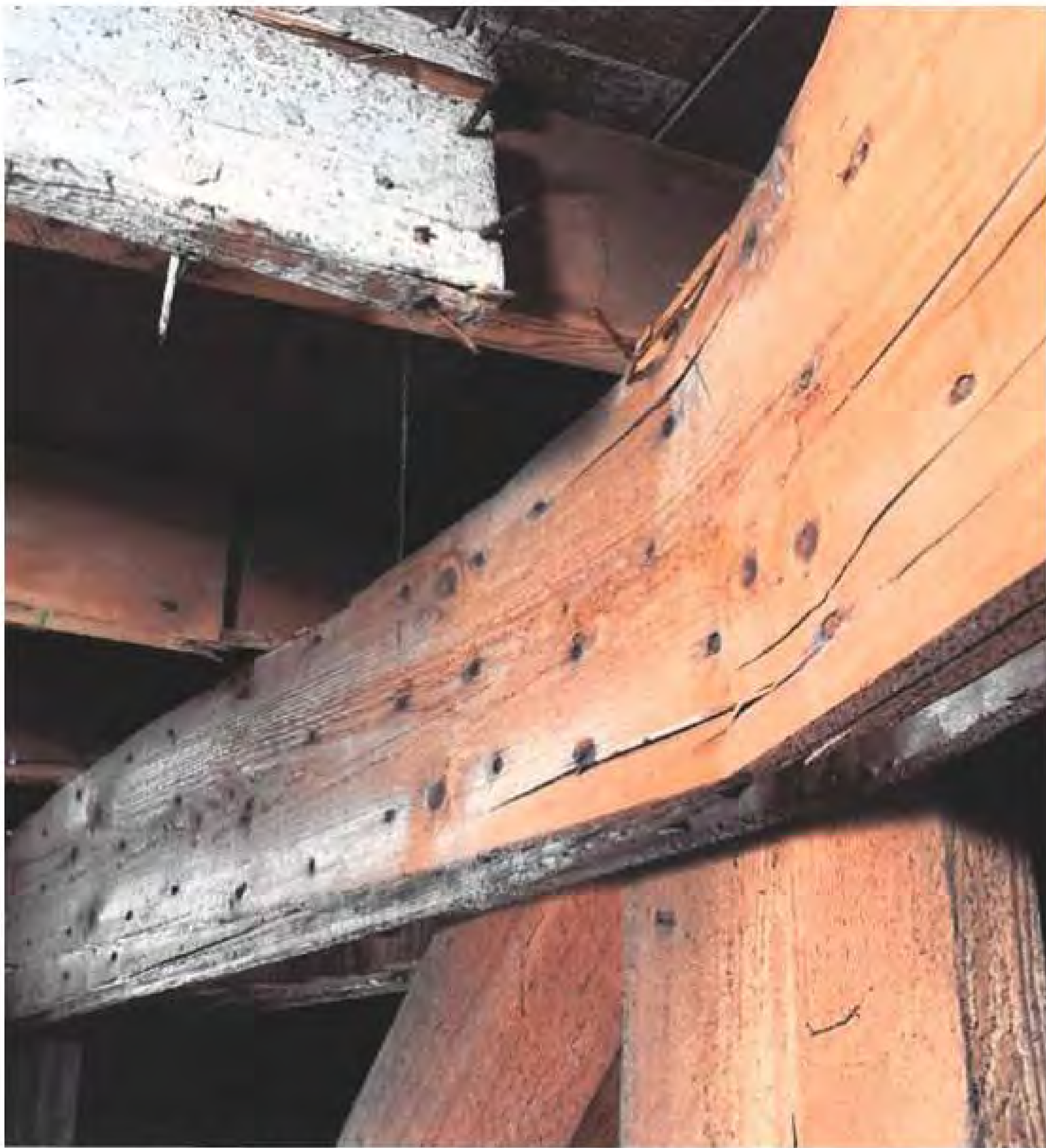
ROOF TRUSS & PURLIN FAILURE
