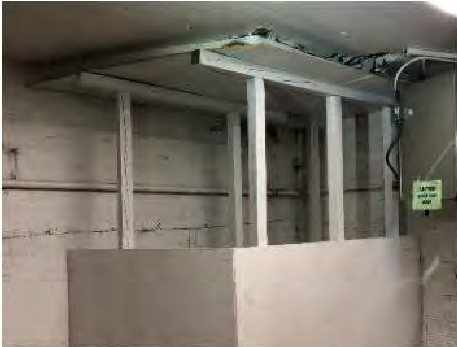
COLLAPSED FIRST FLOOR SLAB
