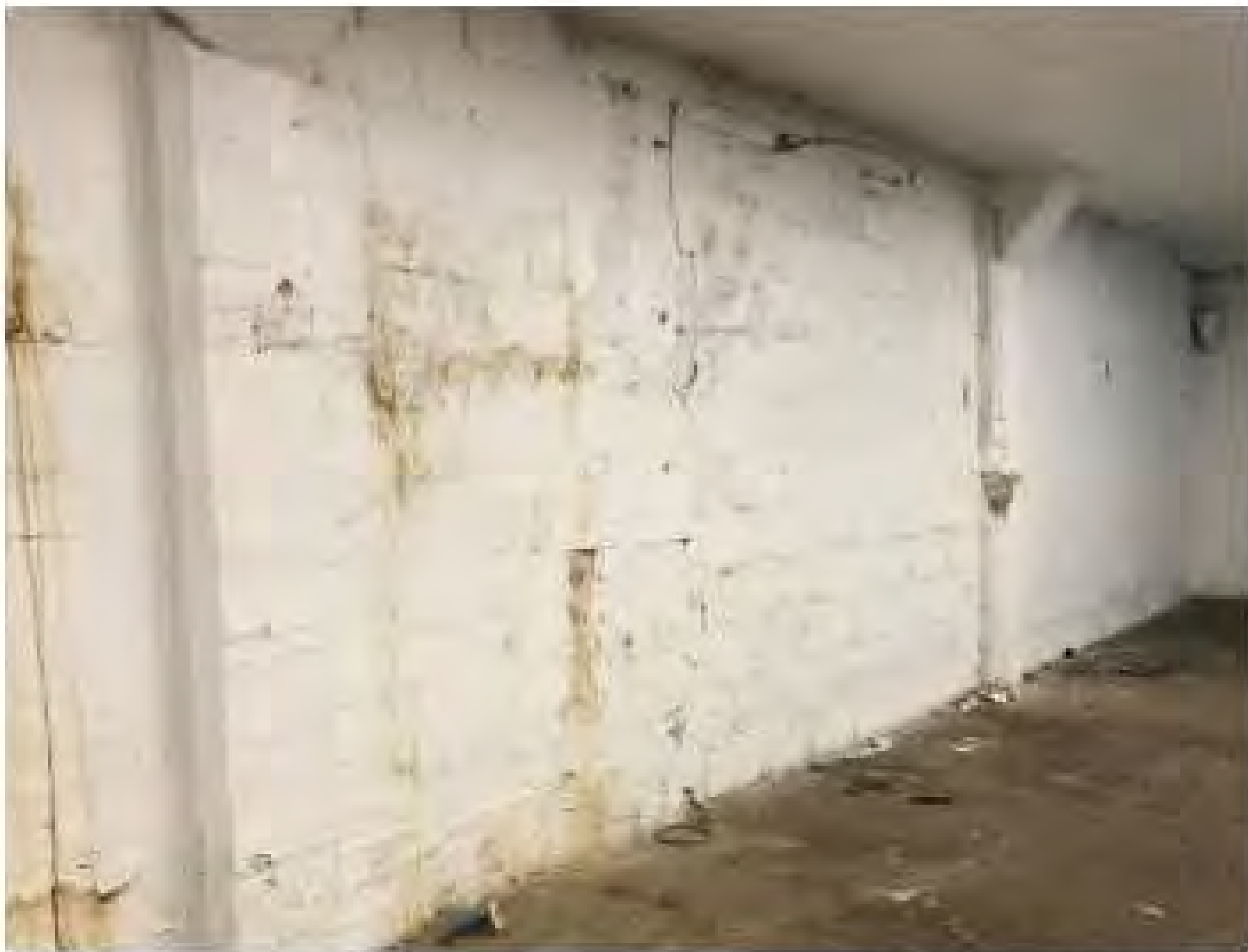
BASEMENT FOUNDATION WALLS DETERIORATED
