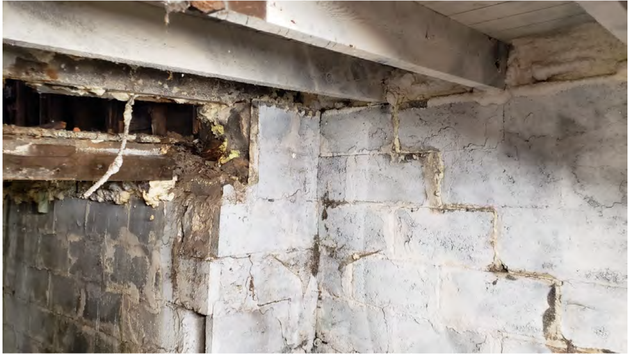
Visible rot where spray foam was removed. Visible step-cracking from the foundation being set on poor footing. Spray foam has been installed in all cavities, promoting rot throughout the structure.
