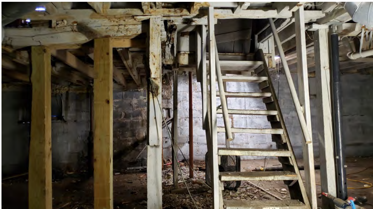
Center stairwell that was added for basement access. Visible main central structural beam both notched for headroom, and broken from neglect. Unsupported floor joists visibly sagging as the house collapses around this centrally located stairwell.
