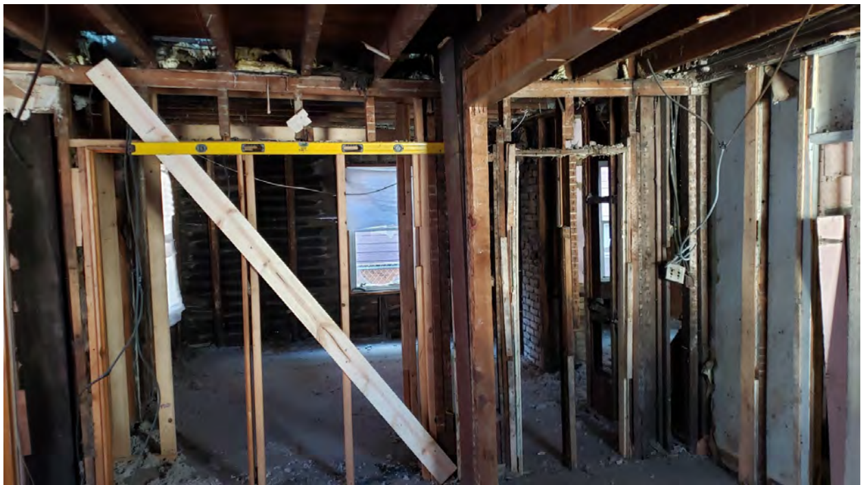
The main interior bearing wall of the original structure's 2nd floor and roof. All load-bearing features were removed or incorrectly altered long ago in both the 1st floor and basement of the building.
