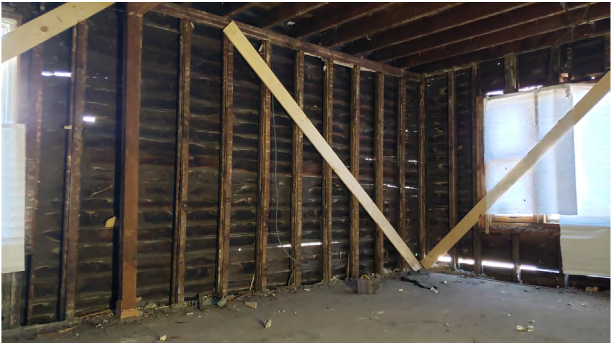
Exterior wall of original structure. The original structure was built without sheathing, which has been a major factor in the many issues this building suffers from.
