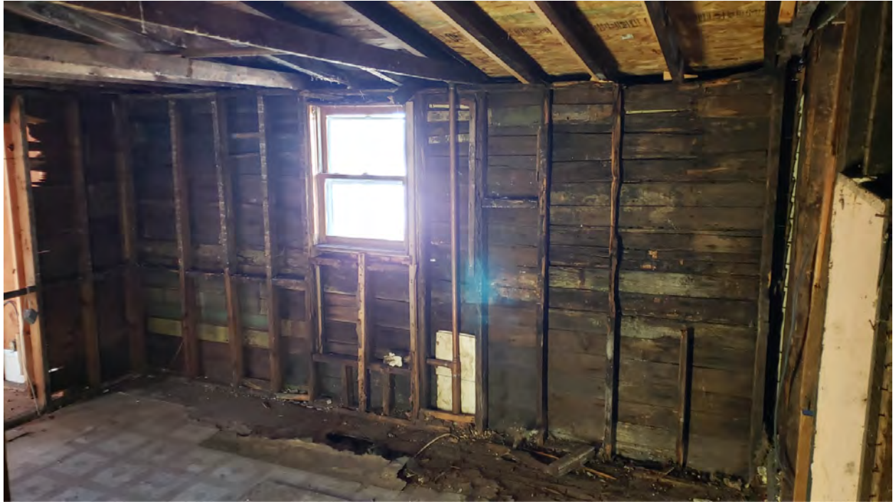
The northwest wall of the building. The structure was neglected for decades, including but not limited to unrepaired roof leaks. This picture shows the rot and collapse of the walls, ceilings, and floor systems on account of a major long-term leak.
