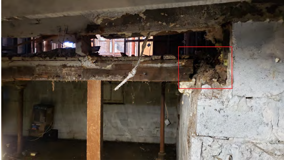
Northwest wall of the basement. The floor systems have been pulled off of the foundation as the center of the house was left unsupported and collapsing after various remodels. Spray foam was added to the outer edge of the building, locking in moisture and promoting rot. Spray foam was removed in the area circled in red, revealing where a structural beam once was located before it rotted away.
