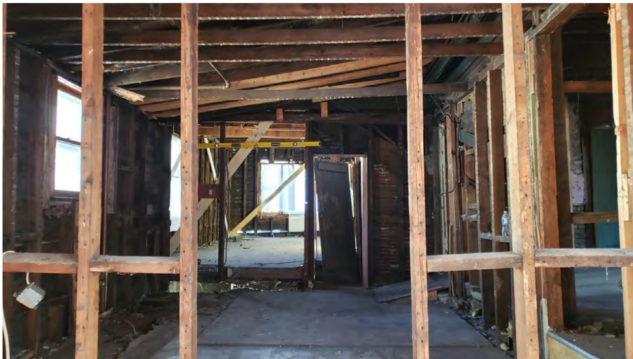
View from rear of building. The southwest addition was built as a lean-to on the southern addition, which led to the 3 rear additions being built at a different height than the original structure.
