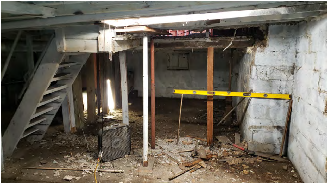
View of basement. Visible collapse of structure around interior basement stairwell addition, and failure of foundation and floor systems. The yellow level in the picture is set at level.
