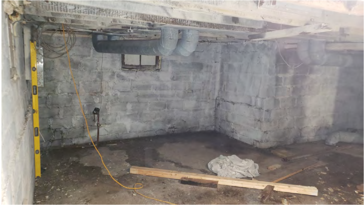
View of northeast wall of basement. The yellow level (at left) is set plumb. The top 5 courses of block were adjusted outward by the original building movers to fit the house upon its delivery to the site. This is a structurally unsound condition that exists throughout the foundation of the original house.
