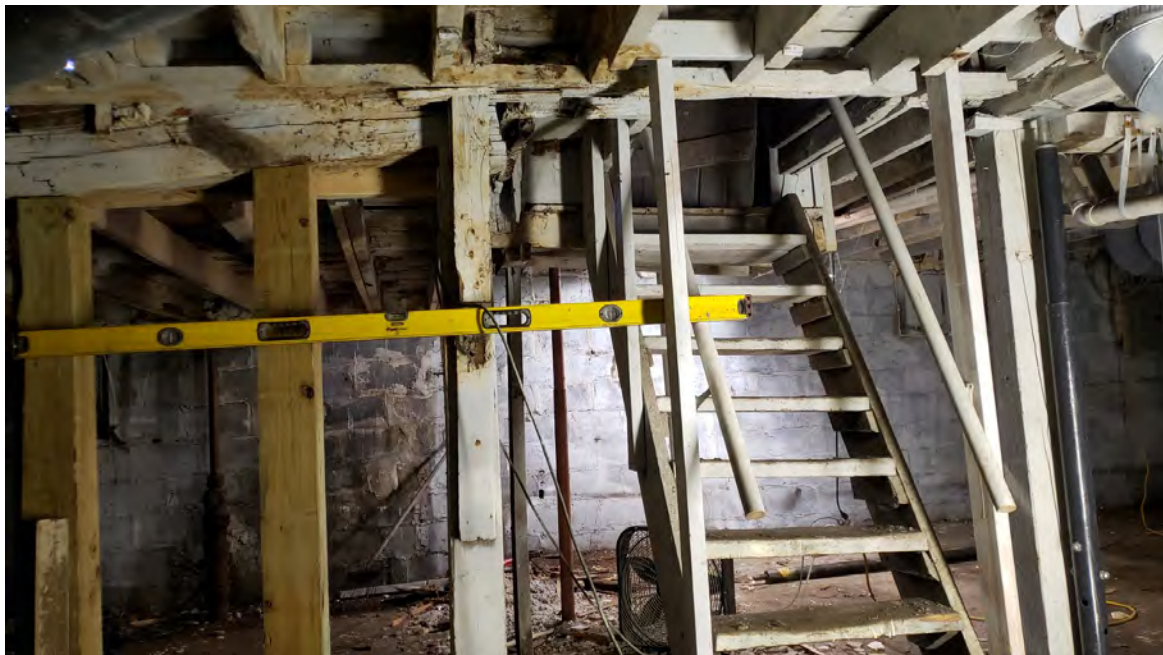
Both intentional and neglectful destruction have played a role in the collapse of the center of the house. Main bearing beams were removed, notched, and left to rot unsupported for decades. The yellow level in the picture is set at level.
