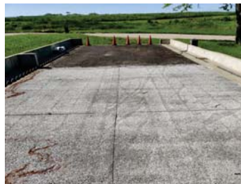
Permeable Pavement Testing Facility - East Side of Madison
