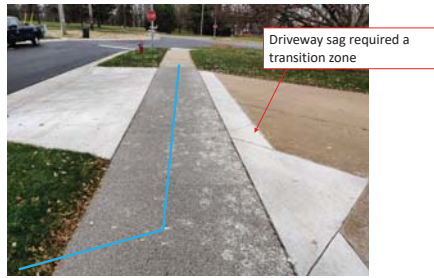
Precast Pervious Panels across driveway
