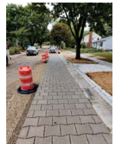
St. Clair Street Pavedrain Section
