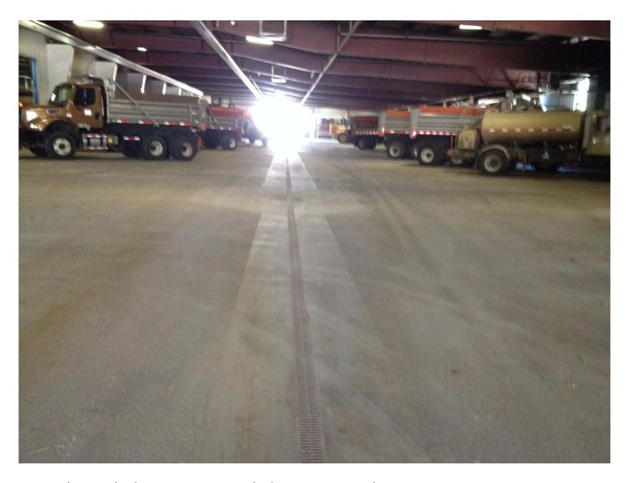
B-1A Indoor vehicle storage – trench drain connected to sanitary sewer
