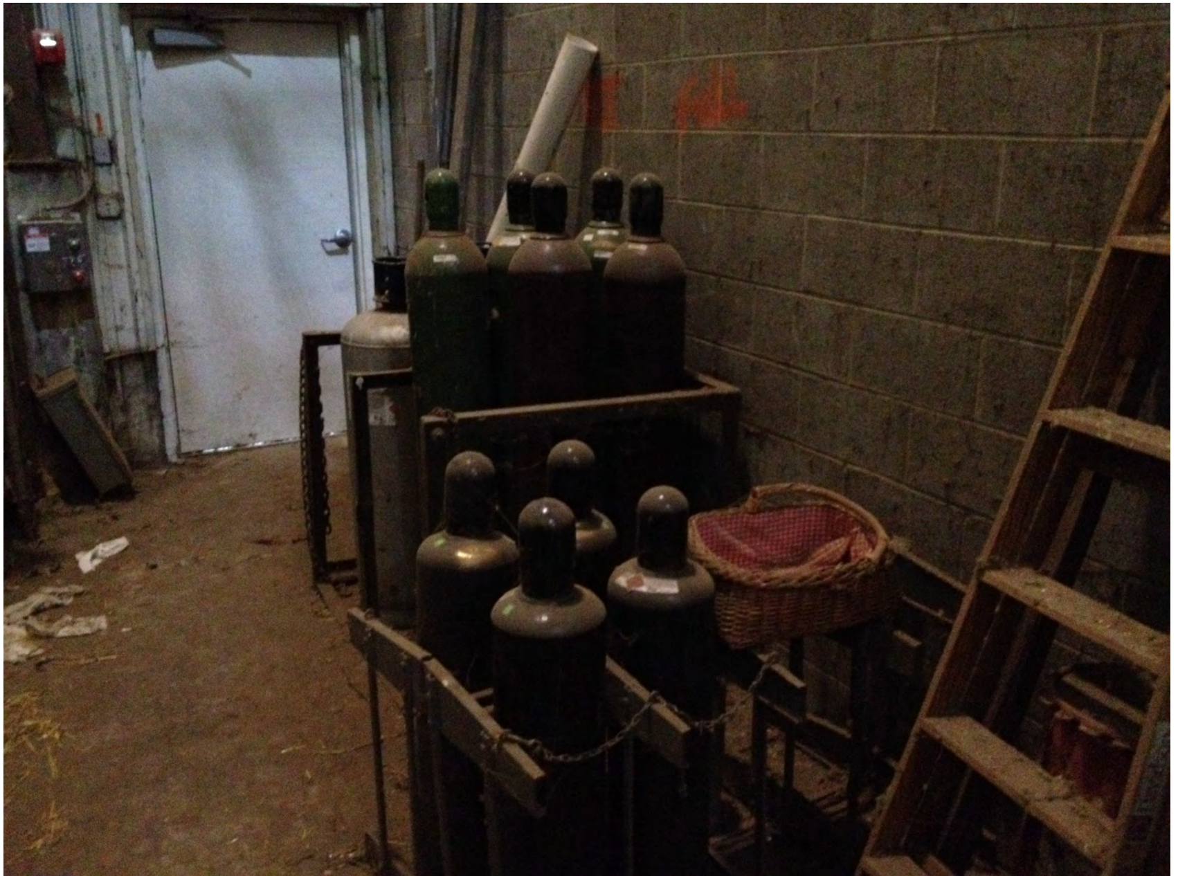
B-3B Acetylene Tanks
