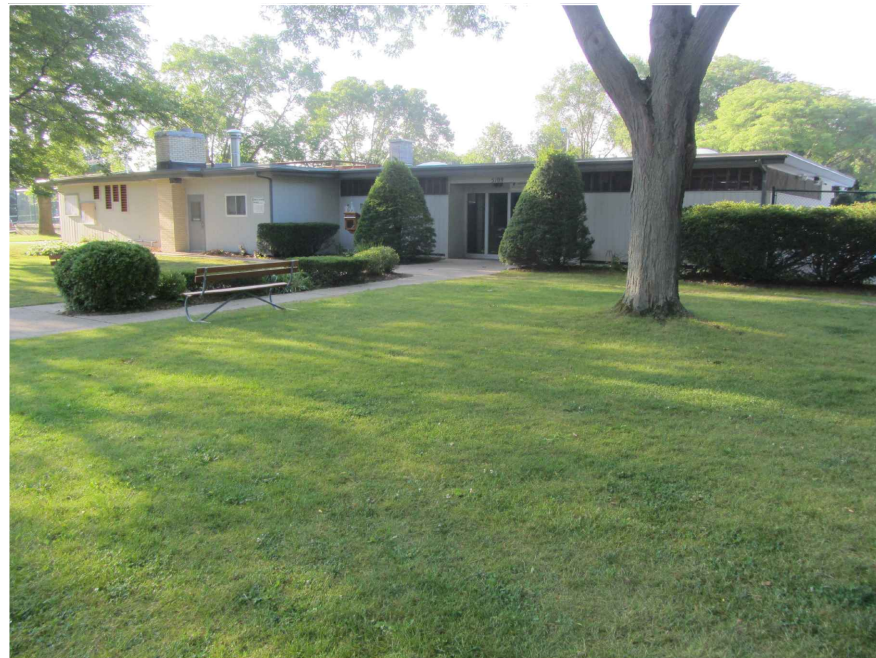
POOL HOUSE FROM NORTH-WEST
