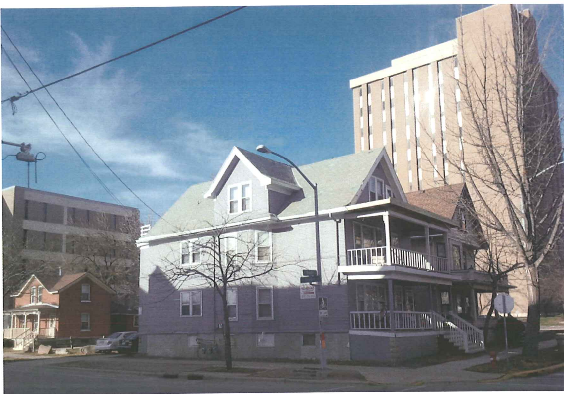
PROJECT SITE FROM THE SOUTHEAST
