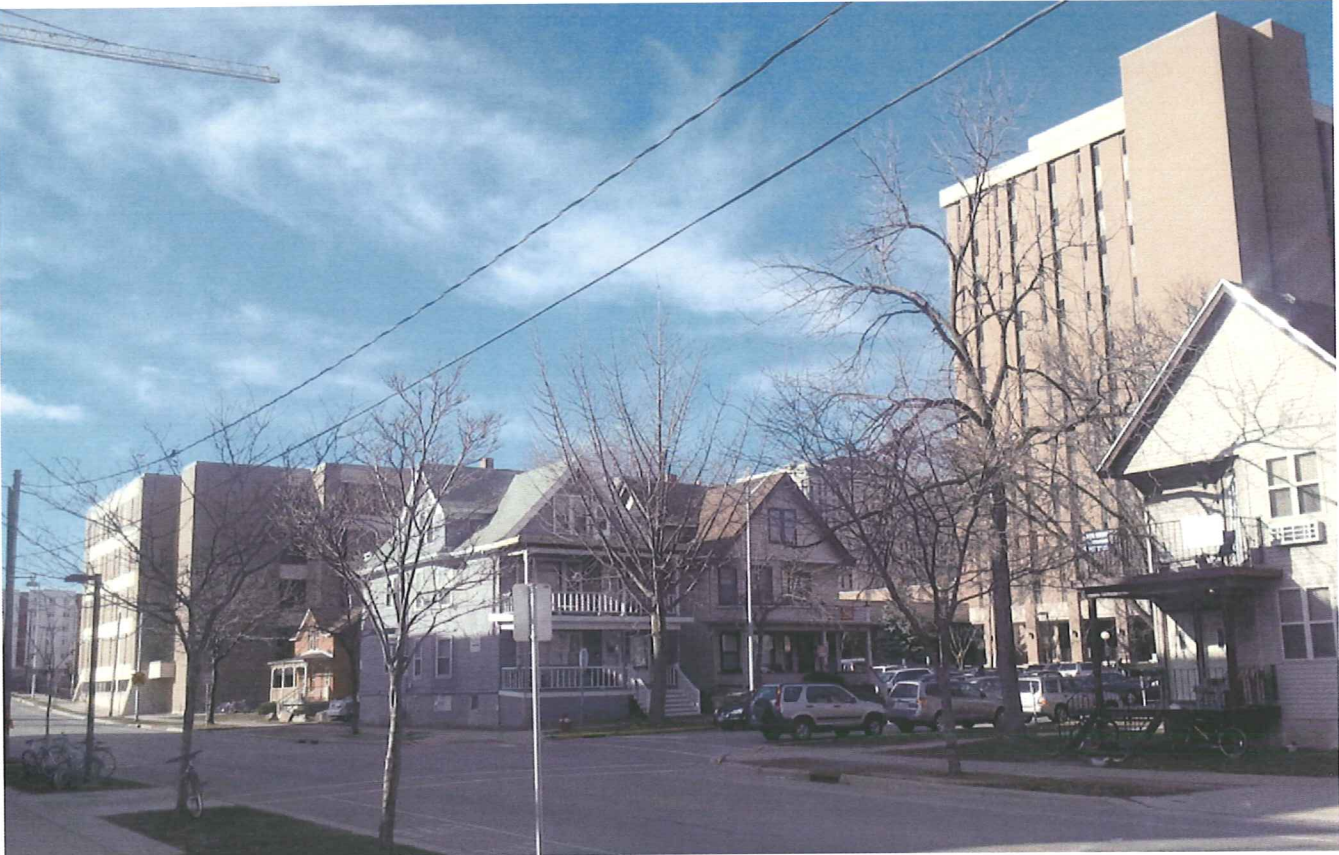
EXISTING STRUCTURES IN CONTEXT - LOOKING WEST DOWN DAYTON
