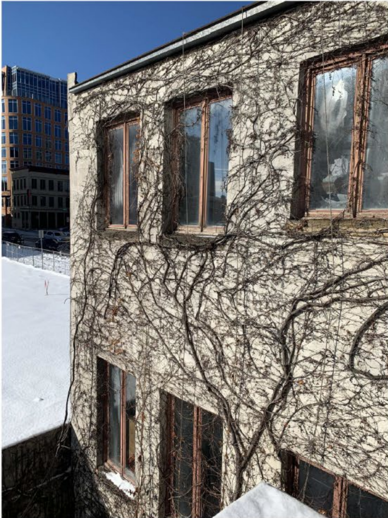
EXISTING CONDITIONS - SOUTHEAST WALL
