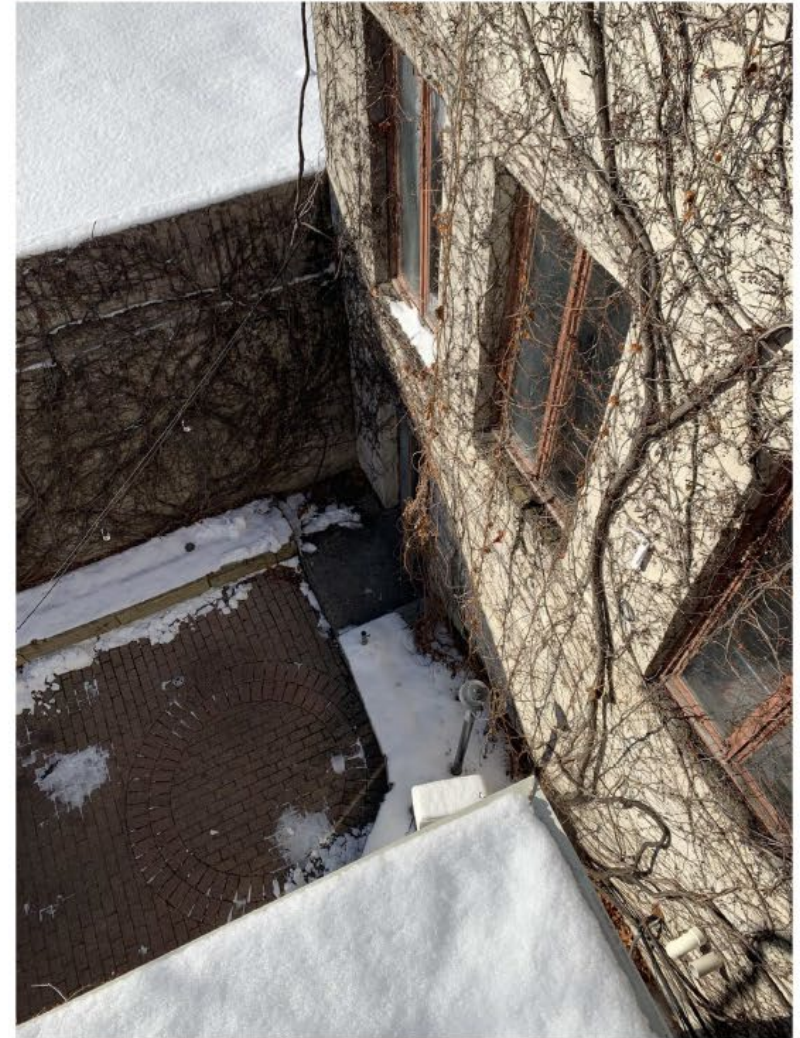
EXISTING CONDITIONS - SOUTHEAST WALL
