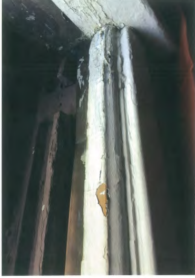
Typical interior of window showing peeling paint, damaged glazing bead, missing hardware, rotted wood, ect...
