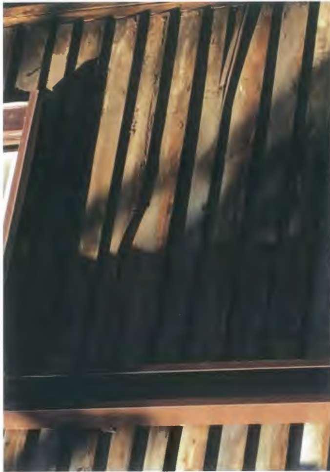
Typical damaged siding panels
