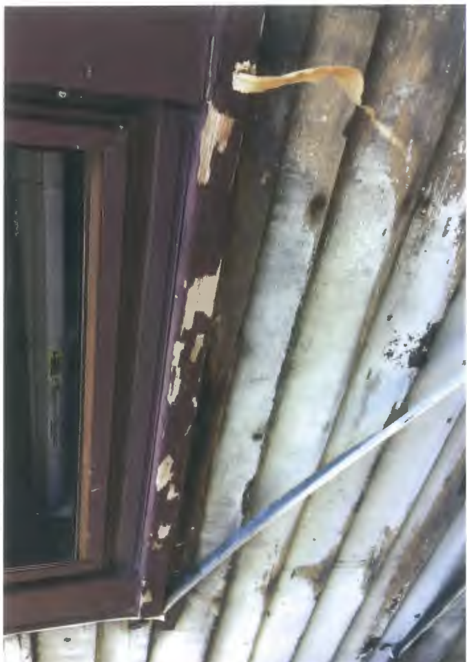
Typical exterior paint peeling and rotten trim and sills on windows
