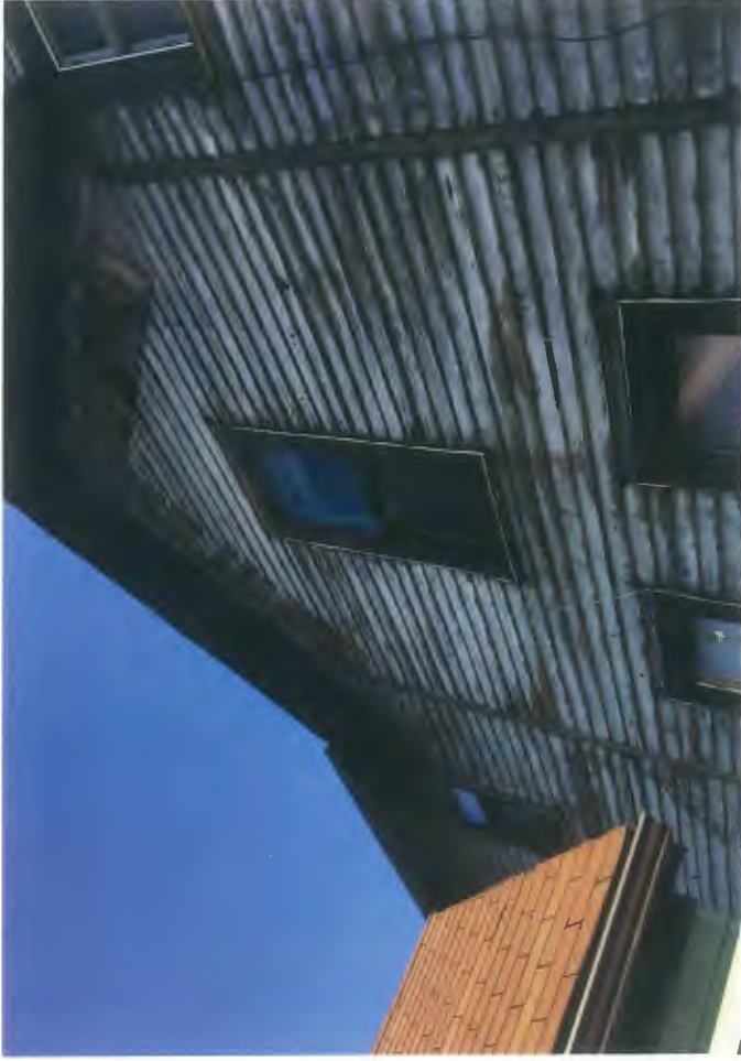
Typical damaged and rotted siding panels
