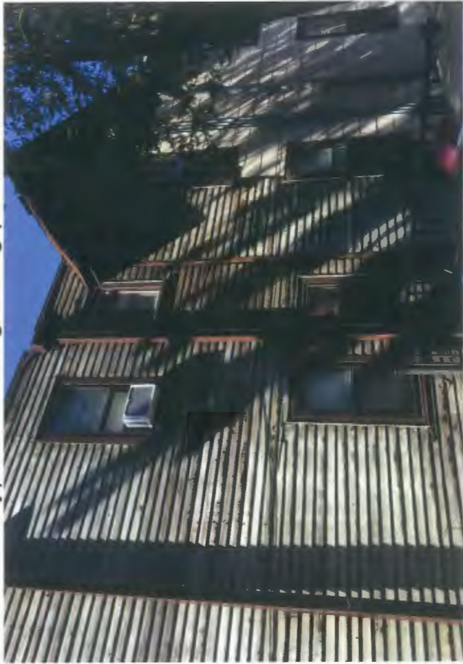
Typical missing siding panels
