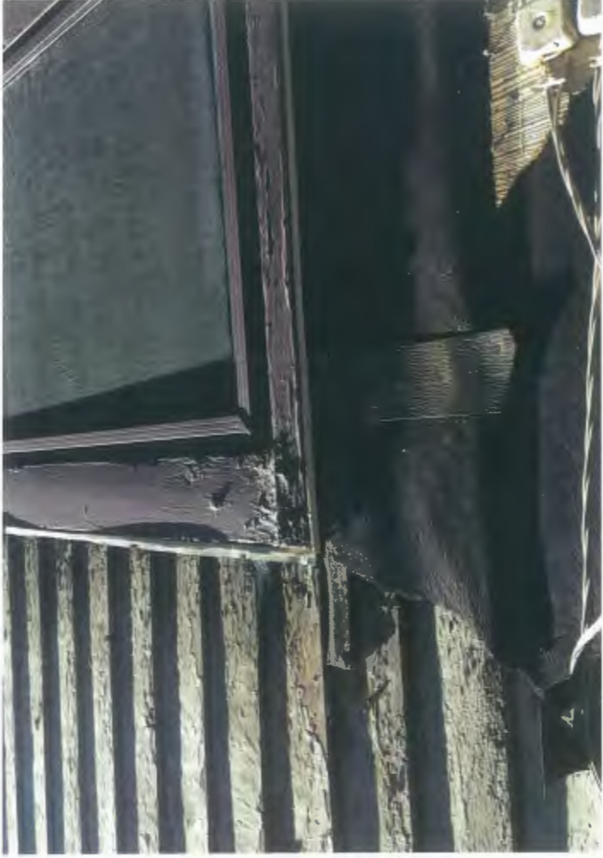
Typical exterior paint peeling and rotten trim and sill on windows
