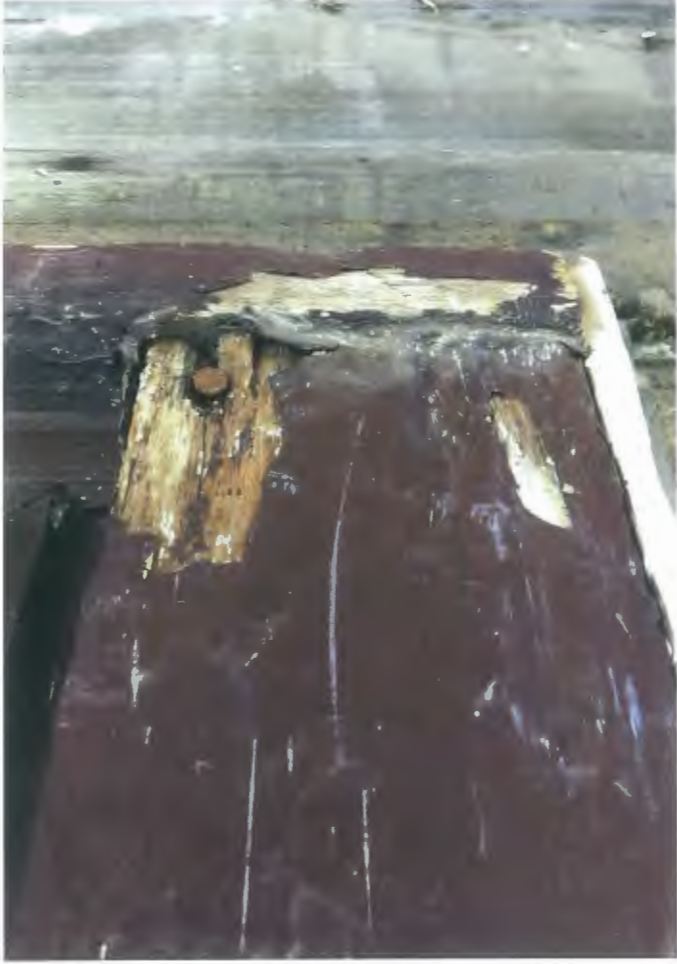
Typical exterior paint peeling and rotten trim and sill on windows
