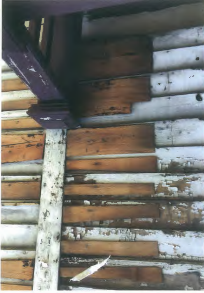
Typical areas of patched siding to conceal damage or missing siding
