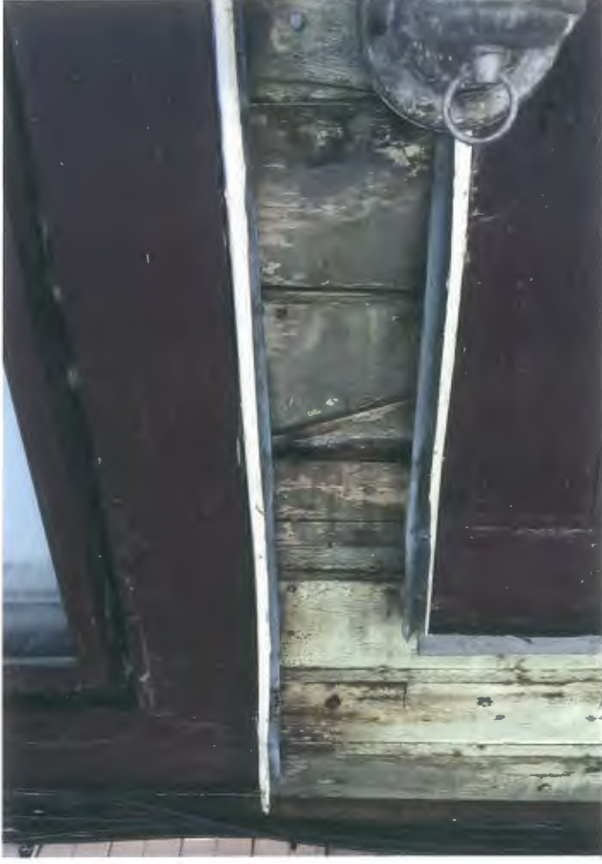
Typical areas of patched, rotted, and missing siding panels
