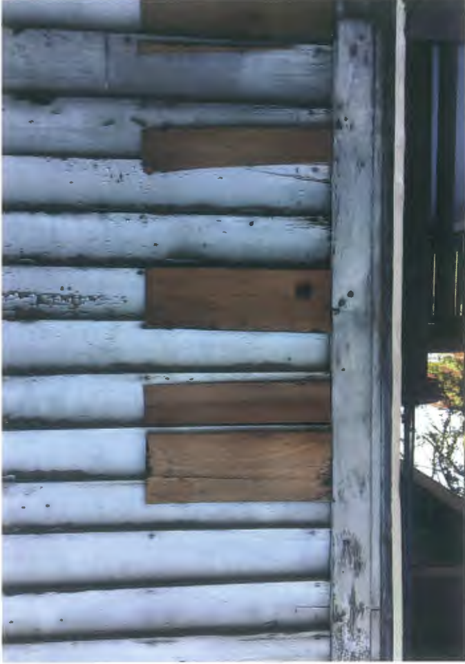
Typical areas of patched, rotted, and missing siding panels
