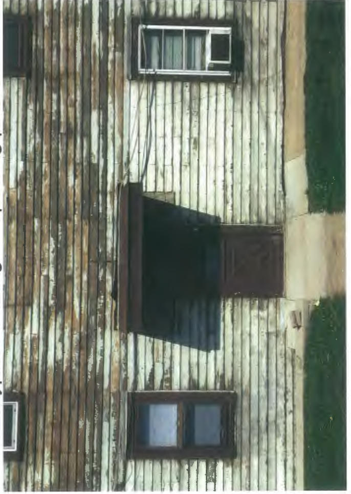
Typical missing and peeling paint
