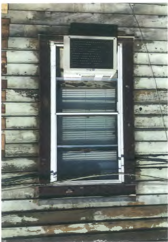
Typical exterior paint peeling and rotten trim and sills on windows
