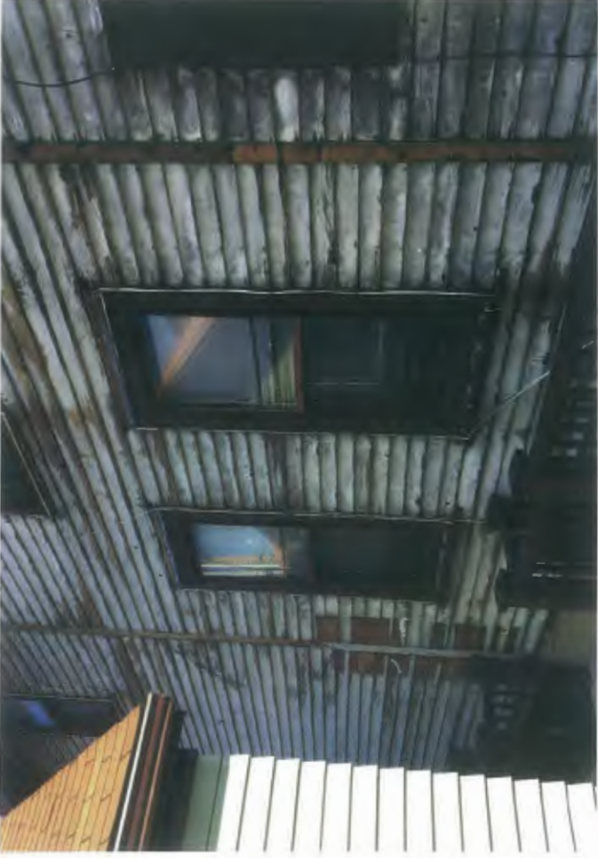
Typical areas of patched siding to conceal damage or missing siding
