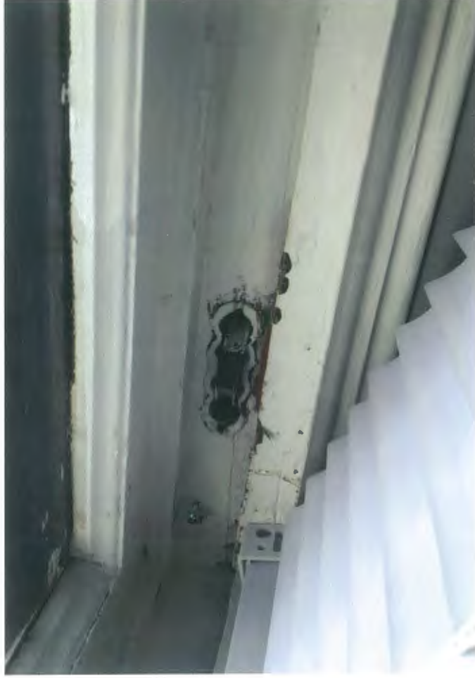
Typical interior of window showing peeling paint, damaged glazing bead, missing hardware, rotted wood, ect...
