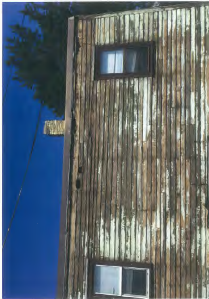
Typical missing siding panels
