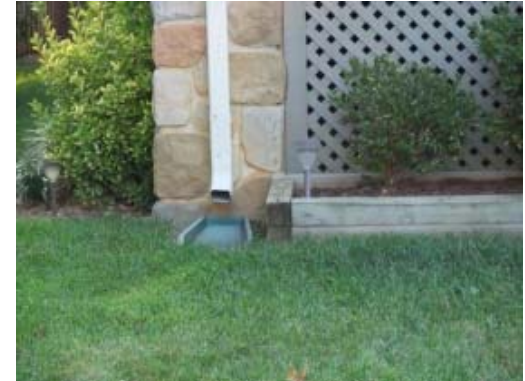
Downspout Disconnection
