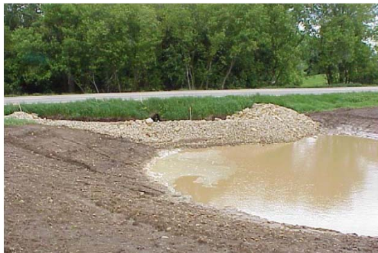
Construction Site Erosion Control
