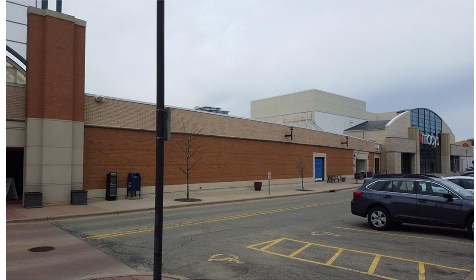
EXISTING EXTERIOR WITH PHASE 1 IN THE BACKGROUND
