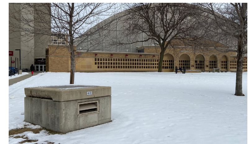
CAMP RANDALL MEMORIAL PARK - SW - MANHOLE
