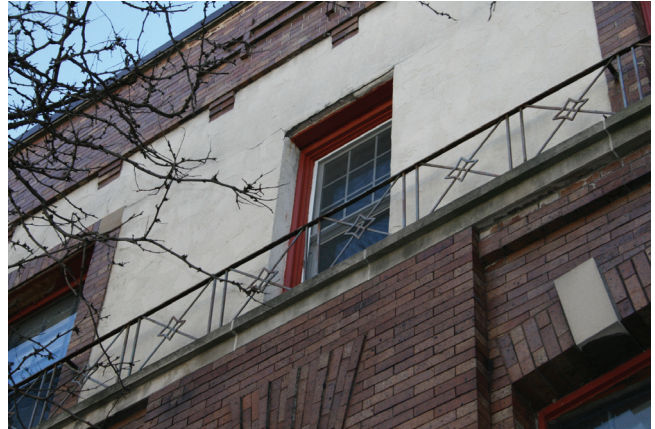
Exterior: View of plaster-coated wall surface
