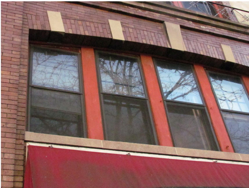
Figure 8. The upper floors of the building typically have original double-hung nine-over-one wood windows, covered by aluminum triple-track exterior storm windows.
