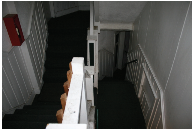
View from third floor down stairs to second floor apartment entrances
