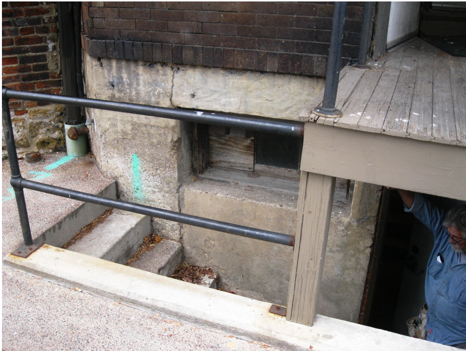
Photo 4 – Stair to basement from Fairchild Street
