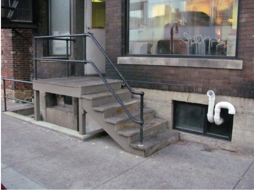
Figure 11. A painted wood stair and platform provide access to a first floor entrance door; there is a sunken well with an entrance door to the basement directly below.
