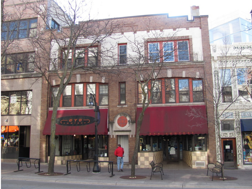
Figure 1. Overall view of the State Street facade.
