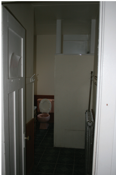
Upper Floor Apartment: Bathroom
