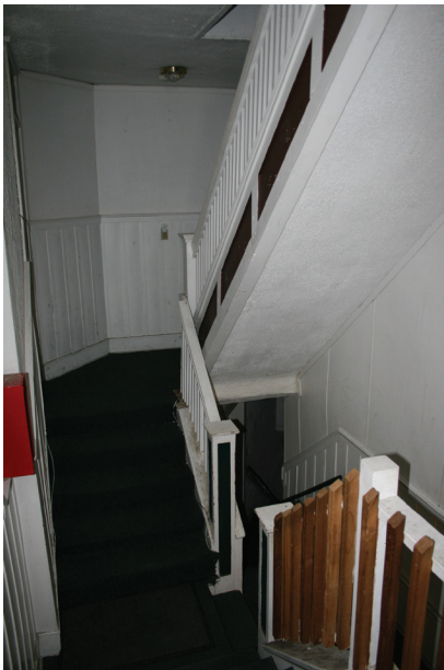
View from third floor toward stair to roof
