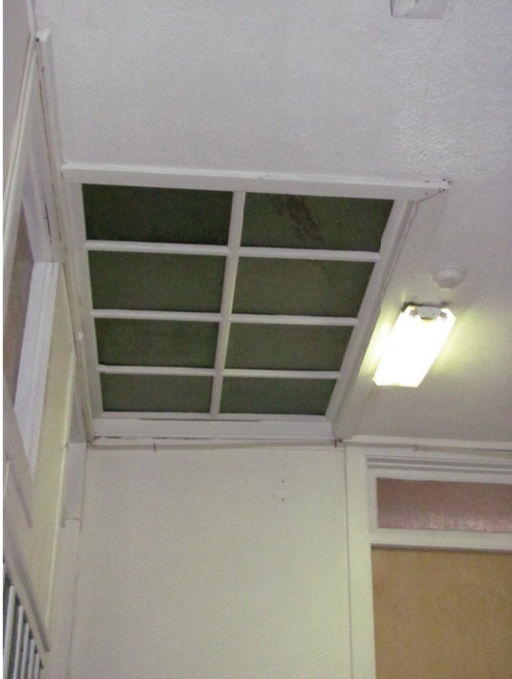
Figure 21. Interior laylight at the third floor corridor.
