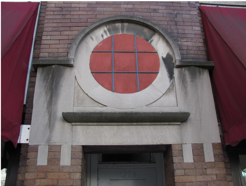
Figure 2. A circular opening above the entrance door to the apartments has been infilled with painted plywood.
