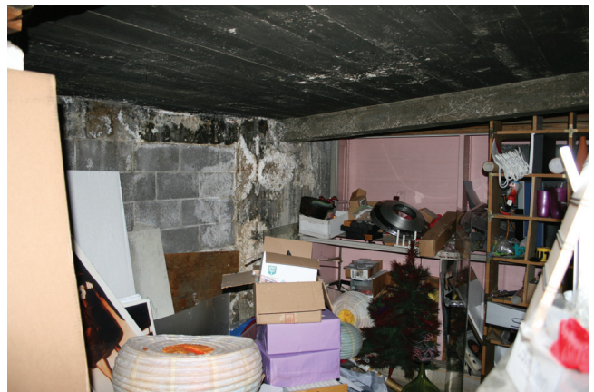
Basement: View of area below an entry ramp to the first floor retail
