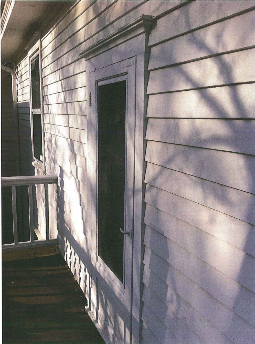
Photo 3: Existing painted wood door screen door (with trim) to exterior porch at stair landing. Proposed screen door to match style, material, and paint color. Proposed exterior trim to match existing door trim style, material, and paint color.
