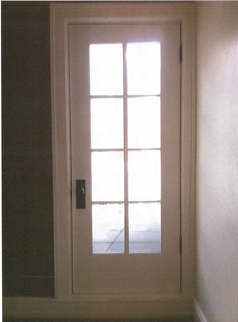
Photo 1: Existing painted wood door to exterior porch at stair landing. Proposed door to be similar (match style, paint color), but only half the proposed door to have divided lite glass.
