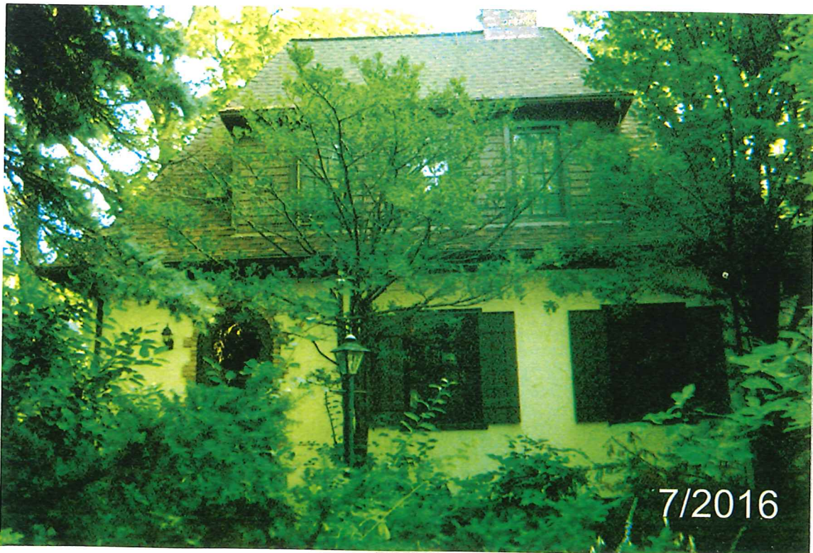
Fig. 4 Street view of 1806 Summit Ave. with new Marvin windows in place (7/2016)
