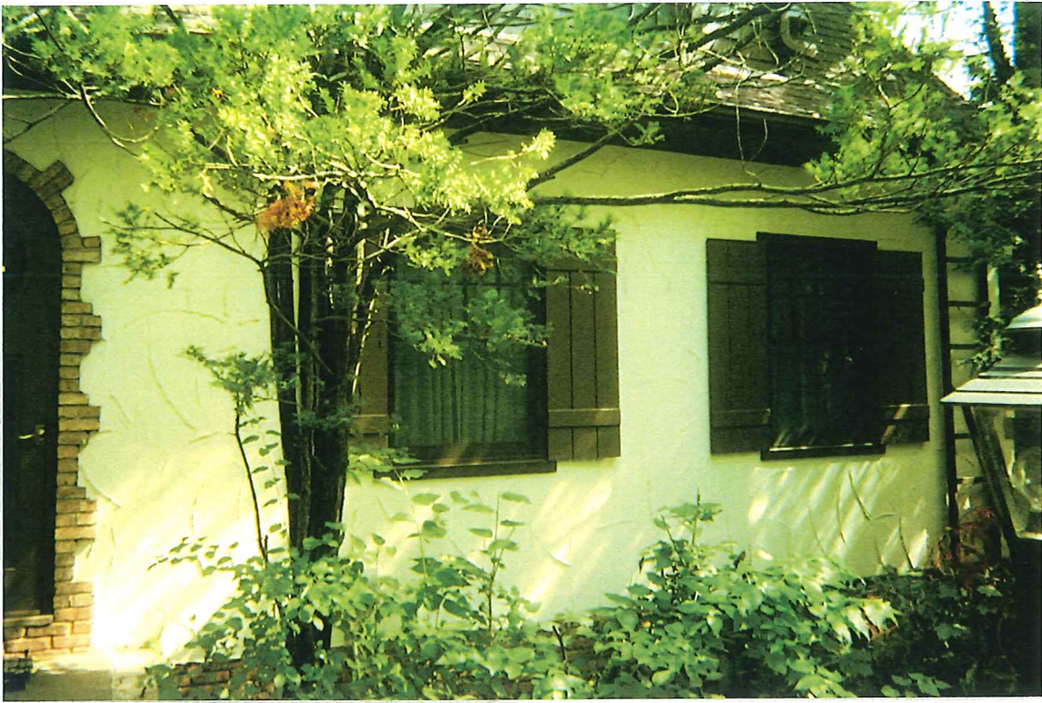
Fig. 5 Exterior (street-side) view of the new Marvin living room windows (7/2016)
