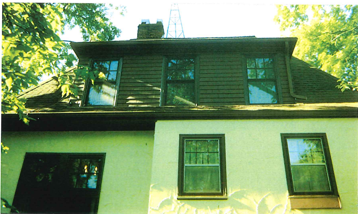
Fig. 9 Exterior view of the three newly installed 2 nd floor Marvin windows (7/2016)
