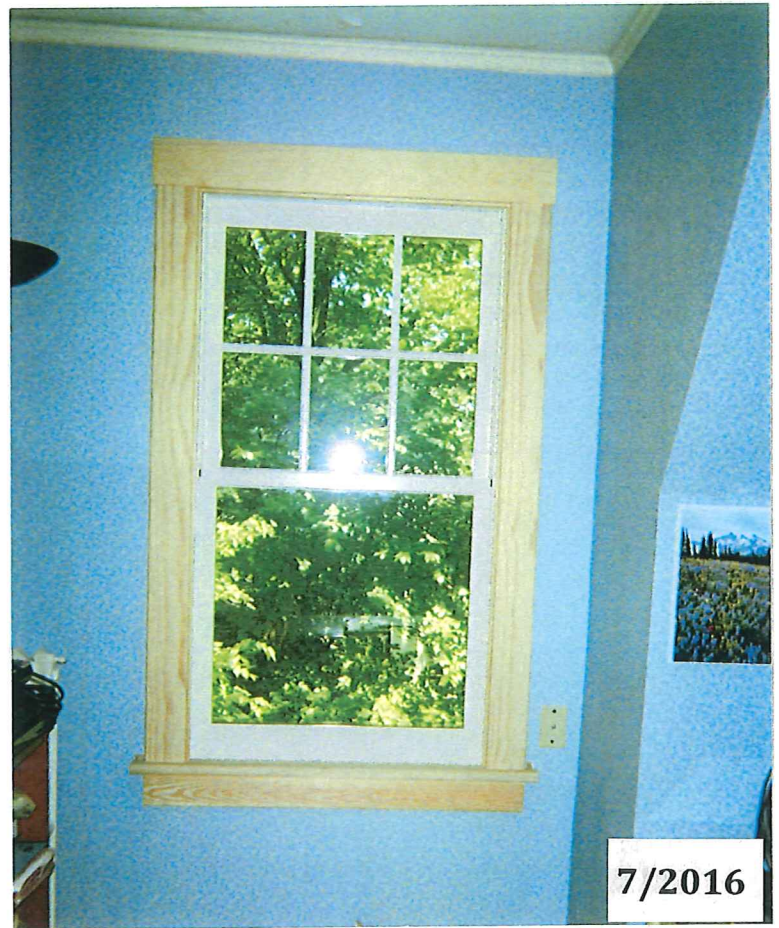
Fig. 8 Interior view of one of the new 2 nd floor north-facing Marvin windows (the replacement of the window shown in Fig. 7)
