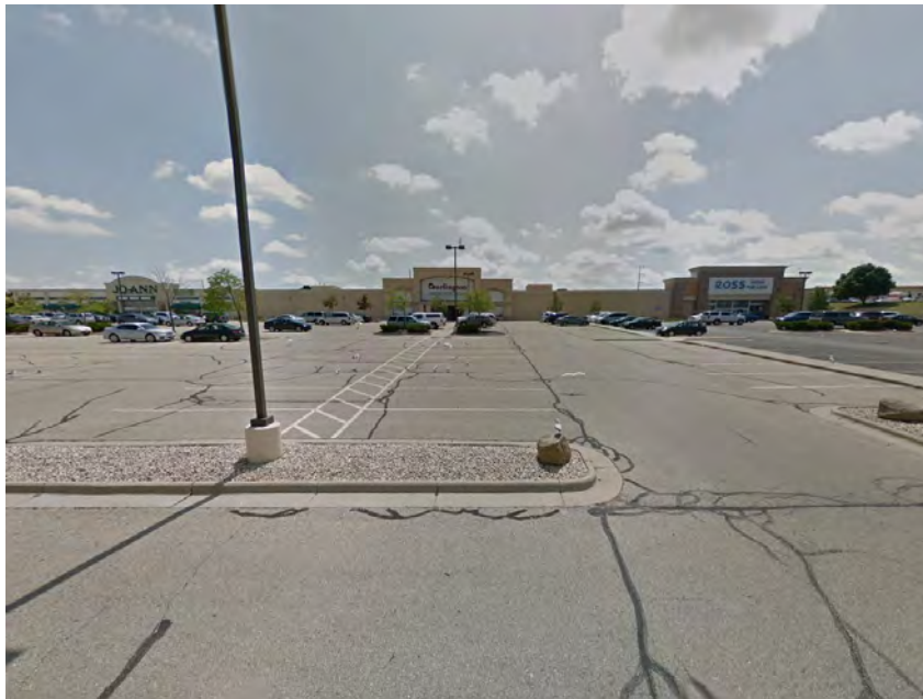
Photo 8: Multi-tenant retail building to south of development via Google (dated August 2018)
