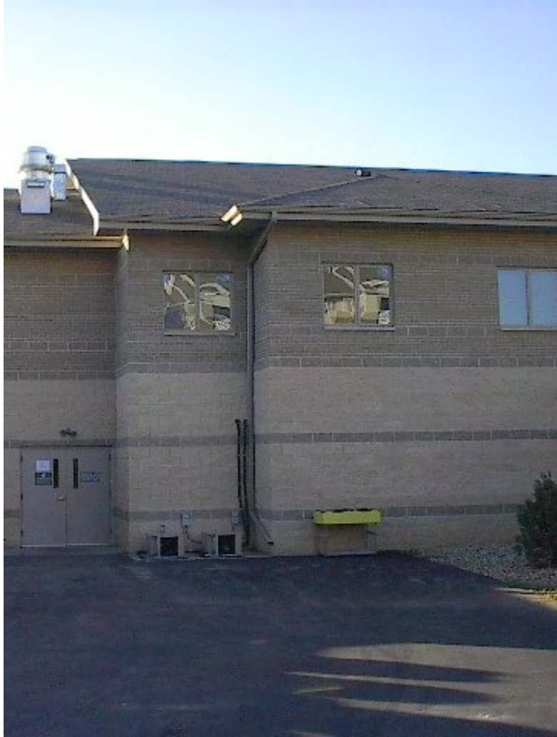
Existing brick and block veneer of Sebring Assisted-Care Residence
