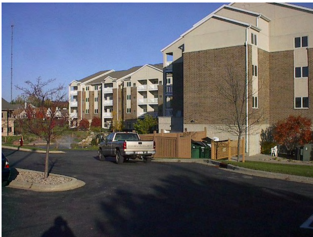
South end of Brookline Congregate Apartments
