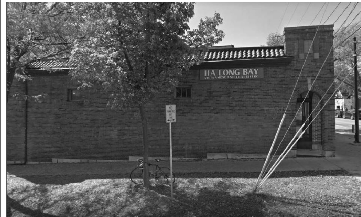
NORTHEAST ORIGINAL ELEVATION PHOTO
