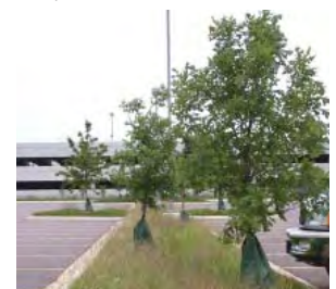
Fig. 3-13: Parking lot with bioswale to filter and absorb runoff. Shade trees reduce heat gain. Tellabs HQ, Naperville, IL.
