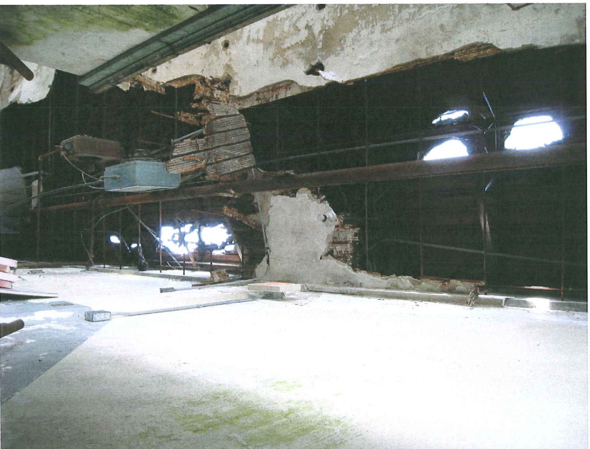
View from Stairwell – Exposed Roof
