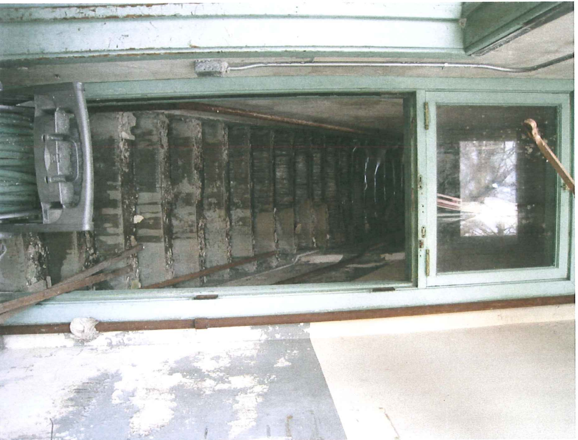
Stairwell from 1 st to 2 nd Floor
