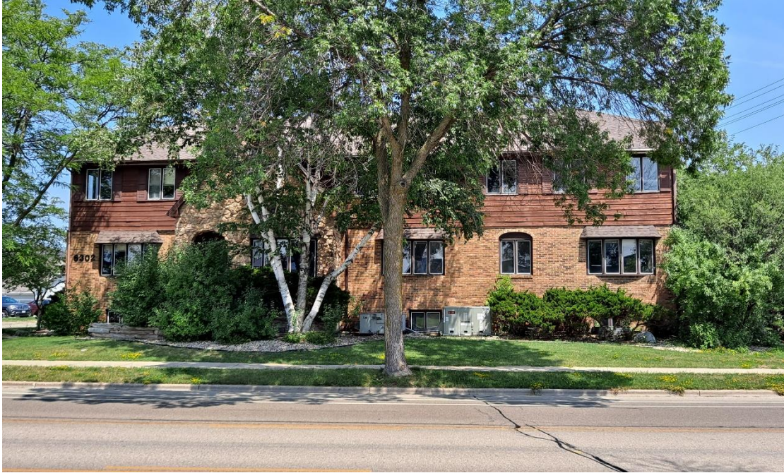
South elevation, view from across Odana Road.
