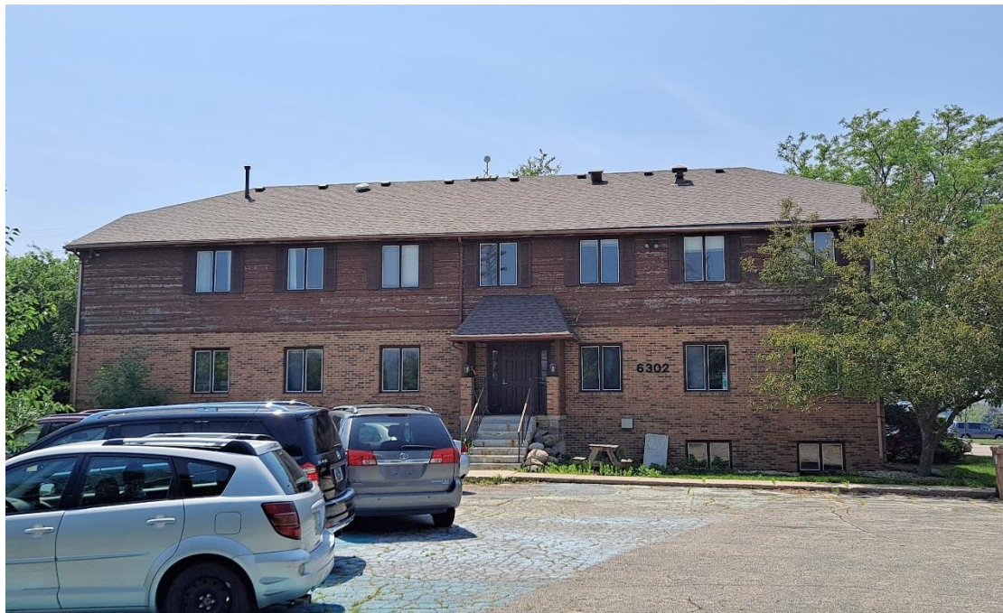
North elevation, view from the parking lot.
