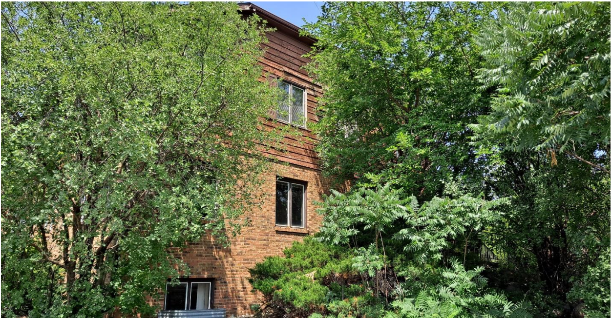
East elevation, obscured by vegetation along the drainage swale, view from the sidewalk.
