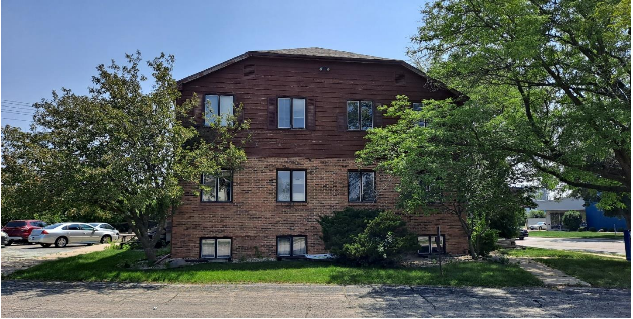
West elevation, view from the parking lot entry.
