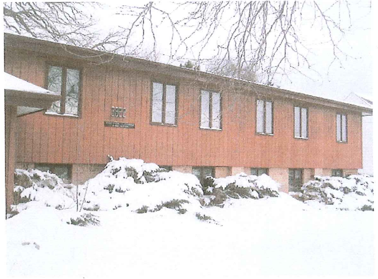
South side of the building (3822 Min. Pt.Rd.)
