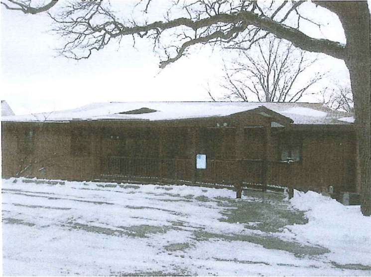
North side of the building (3822 Min.Pt.Rd.)
