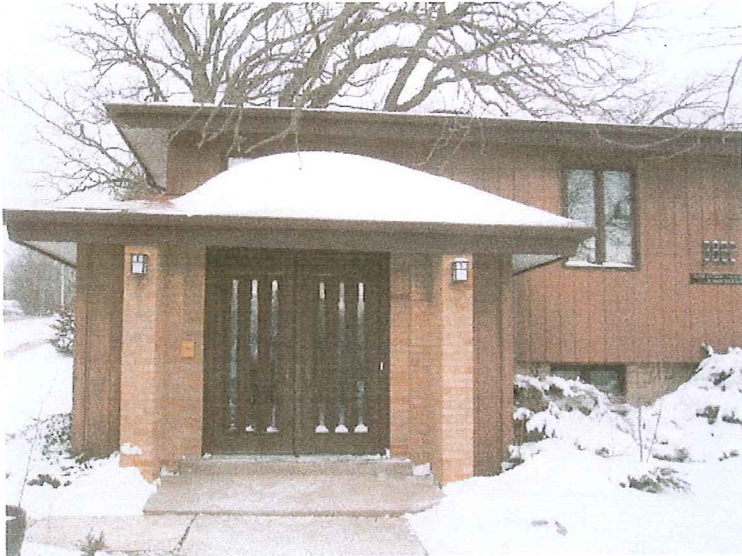
South side of the building (3822 Min. Pt.Rd.)
