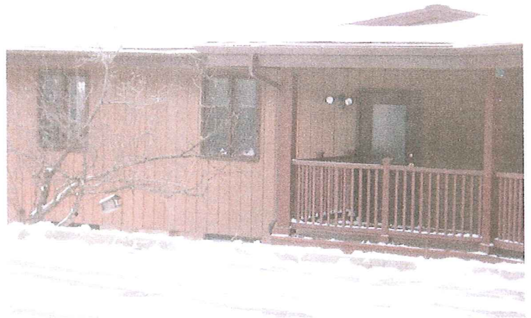
North side of the building (3822 Min.Pt.Rd.)
