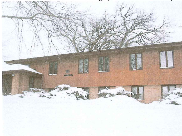
South side of the building (3822 Min. Pt.Rd.)
