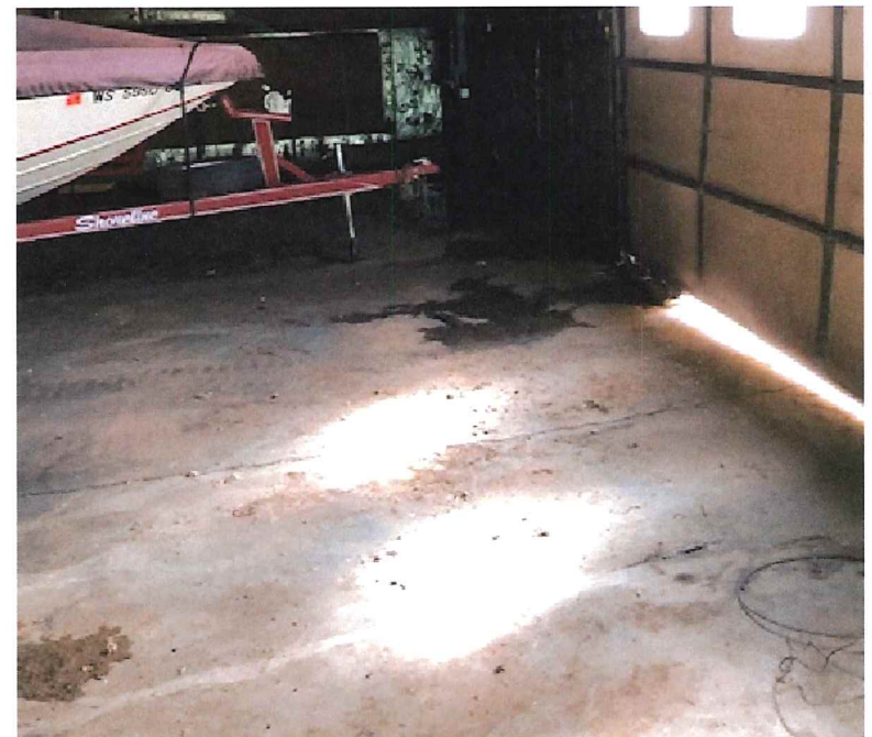
VIEW LOOKING SOUTH AT EAST BUILDING INTERIOR EAST WING
