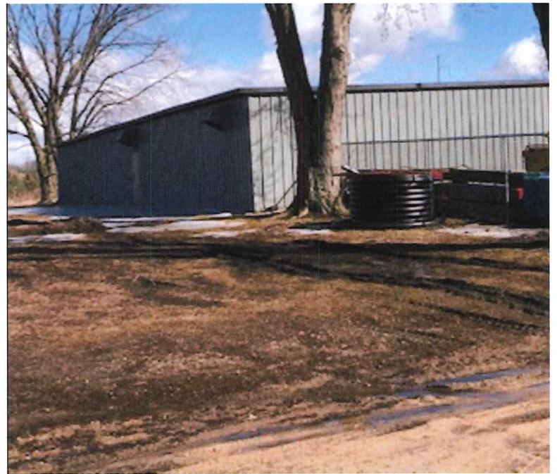
VIEW LOOKING SOUTHEAST AT EAST BUILDING NORTH WALL
