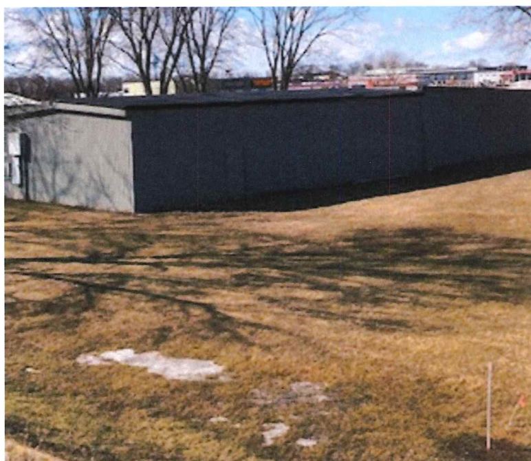
VIEW LOOKING NORTHWEST AT EAST BUILDING EAST WALL
