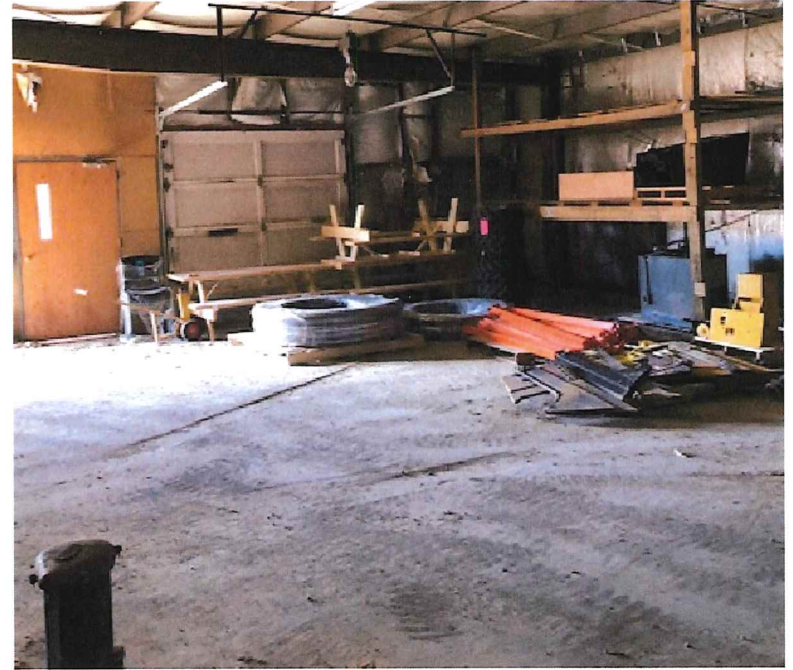
VIEW LOOKING AT EAST BUILDING INTERIOR EAST WING
