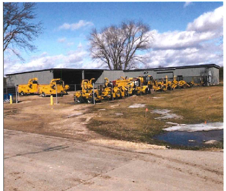
VIEW LOOKING NORTHEAST AT EAST BUILDING EAST/SOUTH WALL
