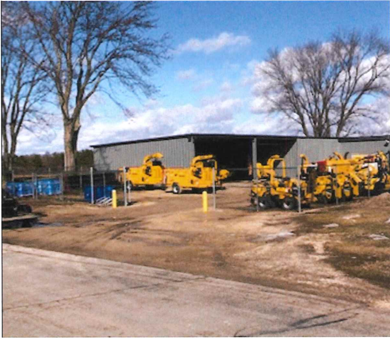
VIEW LOOKING NORTHEAST AT EAST BUILDING EAST WALL
