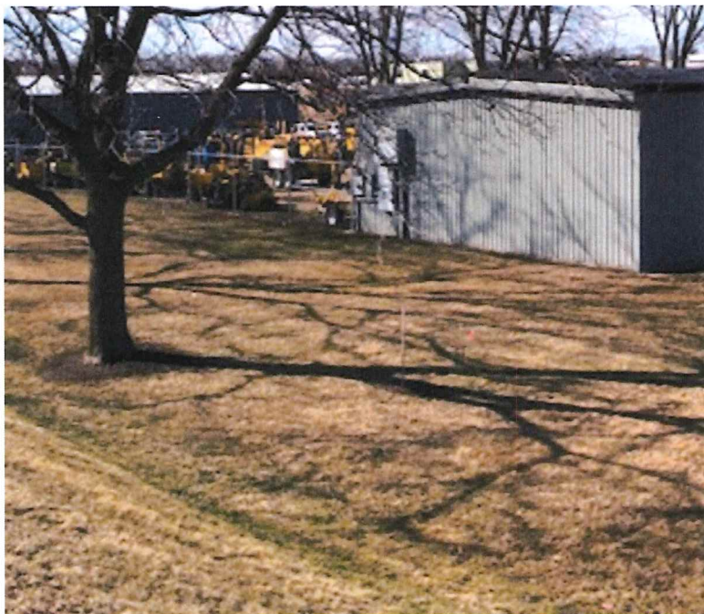
VIEW LOOKING NORTHWEST AT EAST BUILDING SOUTH WALL
