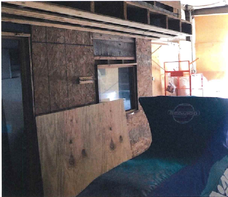
VIEW LOOKING AT EAST BUILDING SMALL ROOM EAST WING
