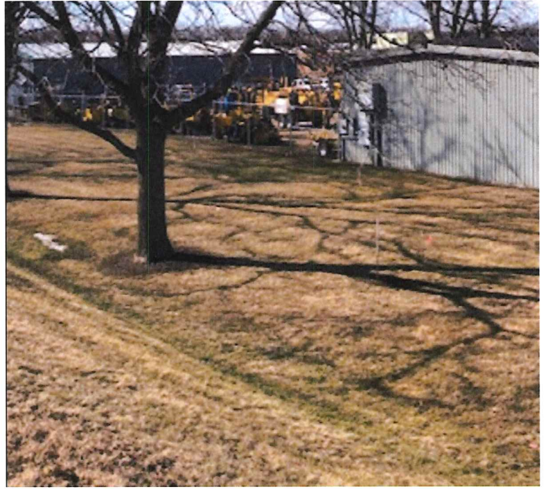
VIEW LOOKING NORTHWEST AT EAST BUILDING SOUTH WALL
