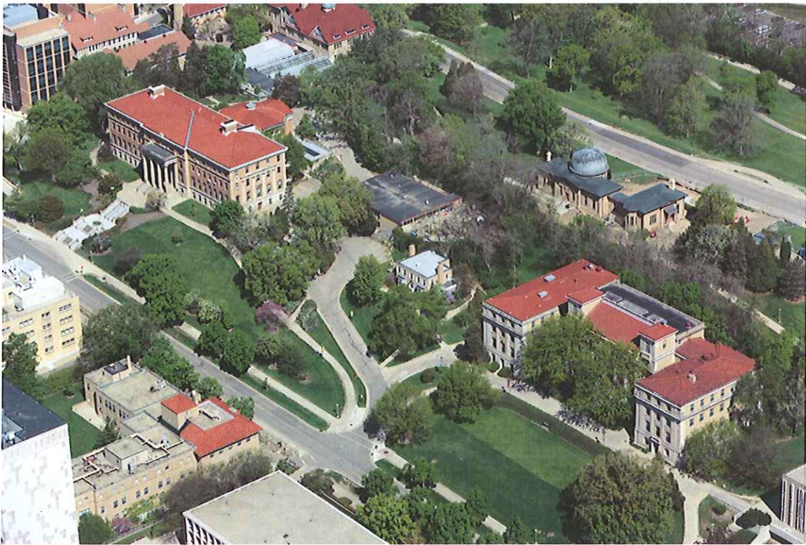
Building Site from above, looking northwest
