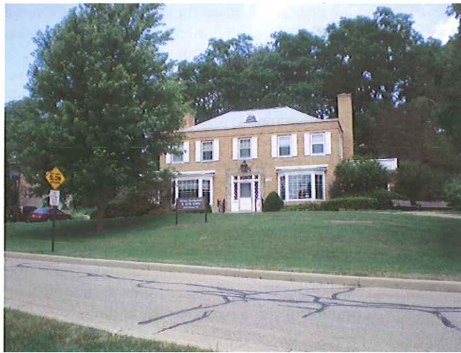
South façade, main elevation
