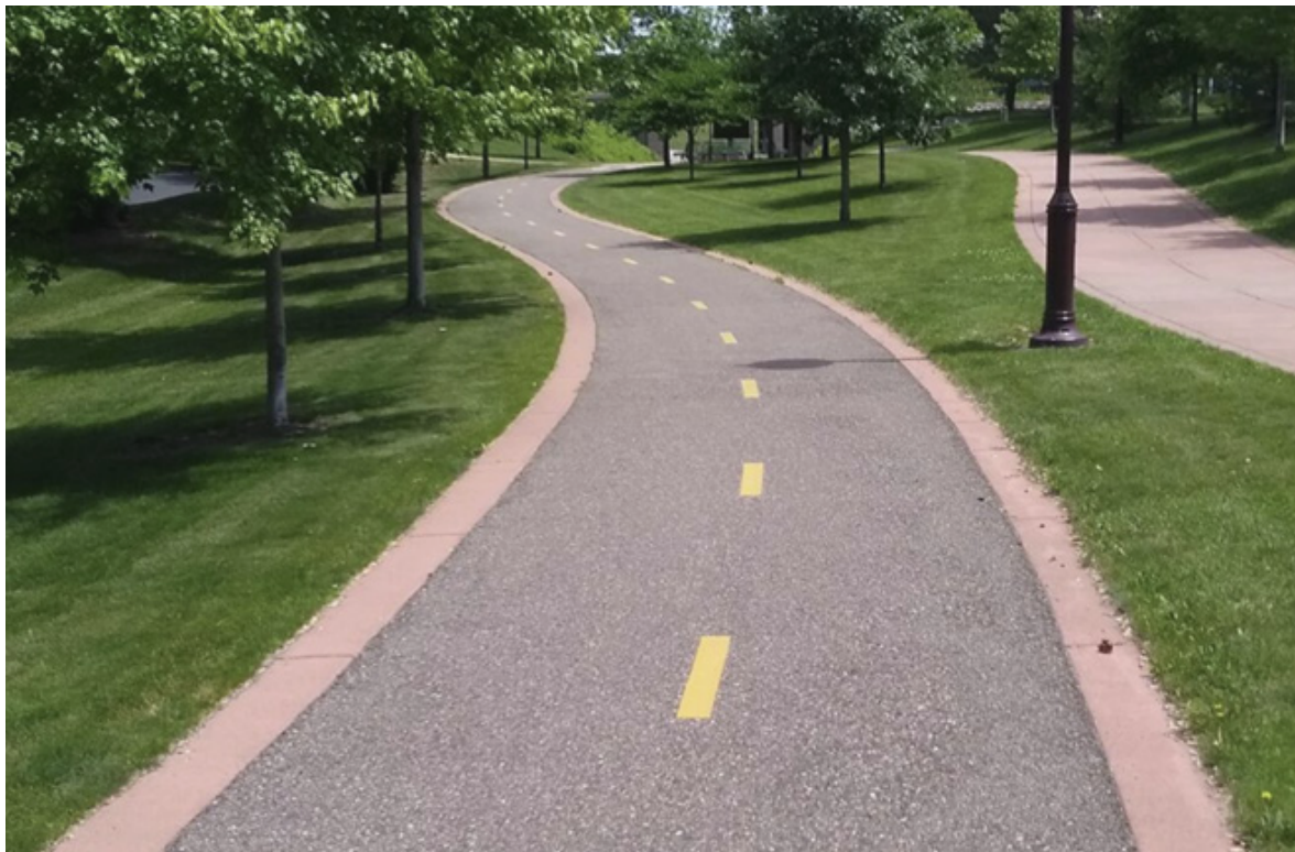
Asphalt path with concrete shoulder and striping
