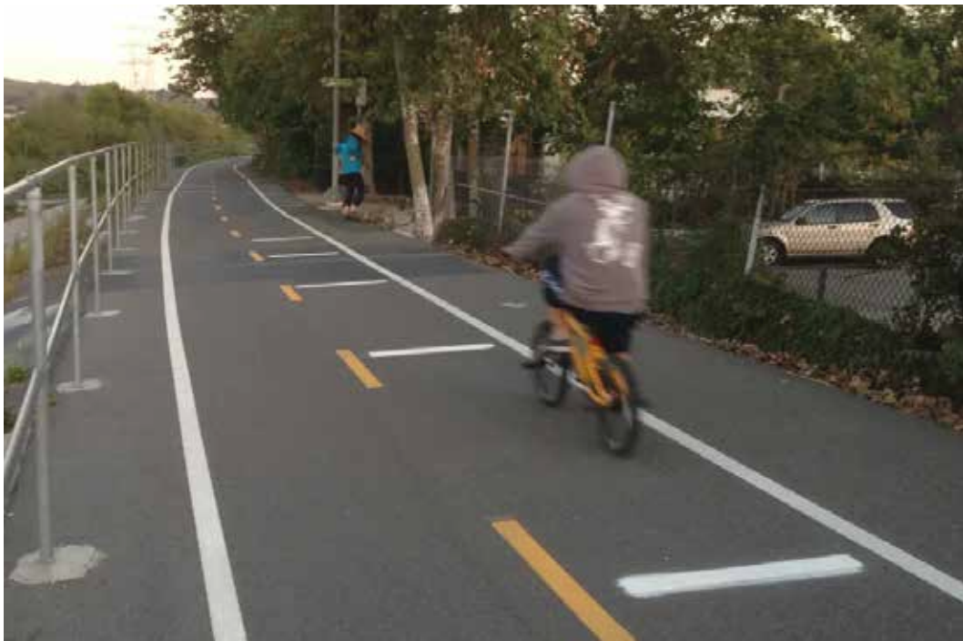
Rumble strips in bike lane before curve
