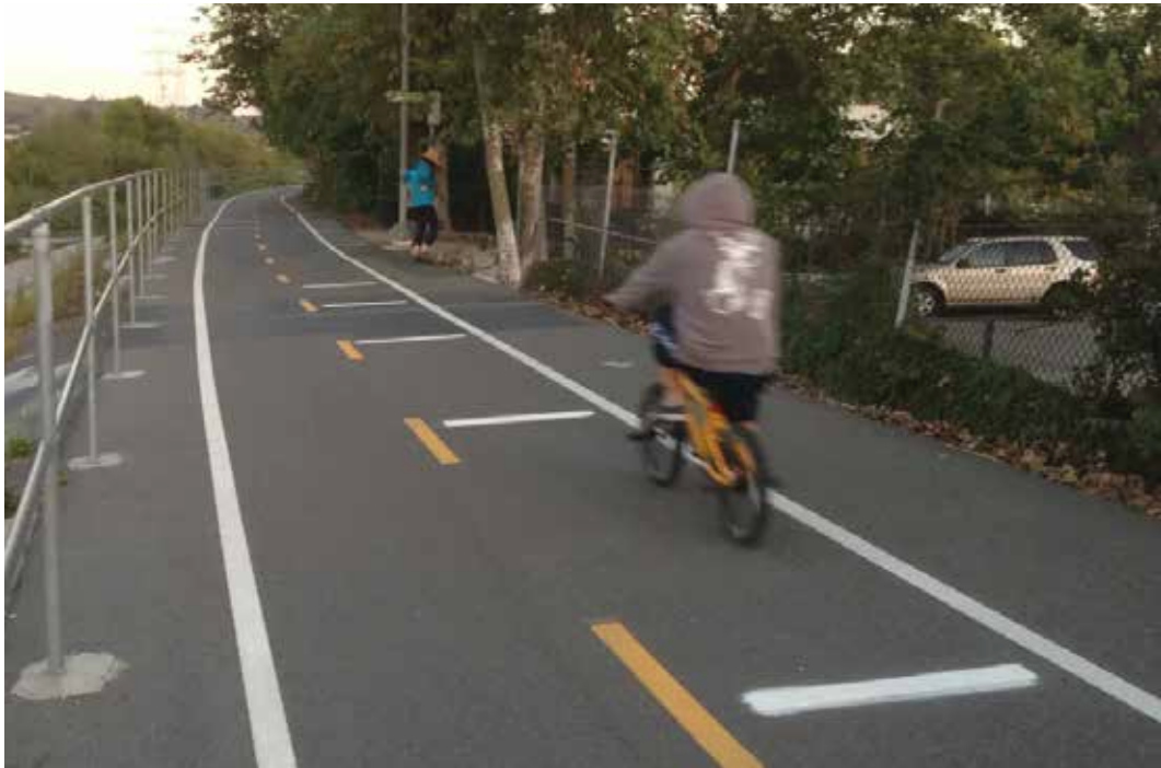
Rumble strips in bike lane before curve
