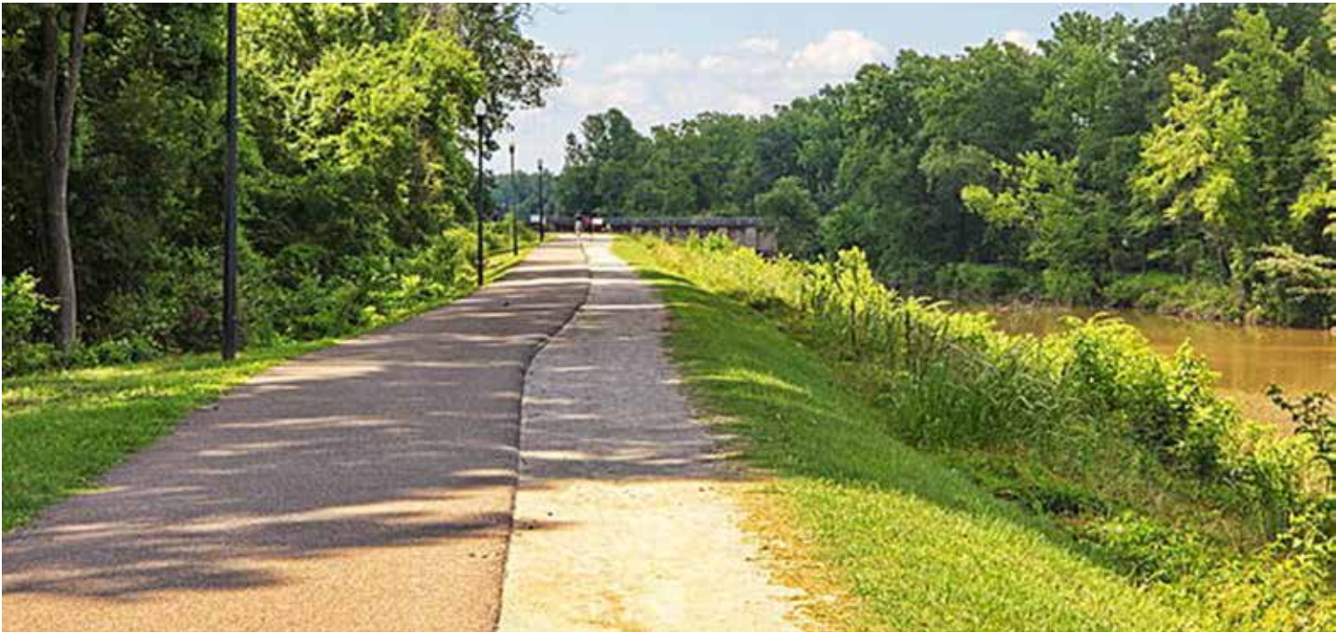
Typical asphalt with aggregate running strip
