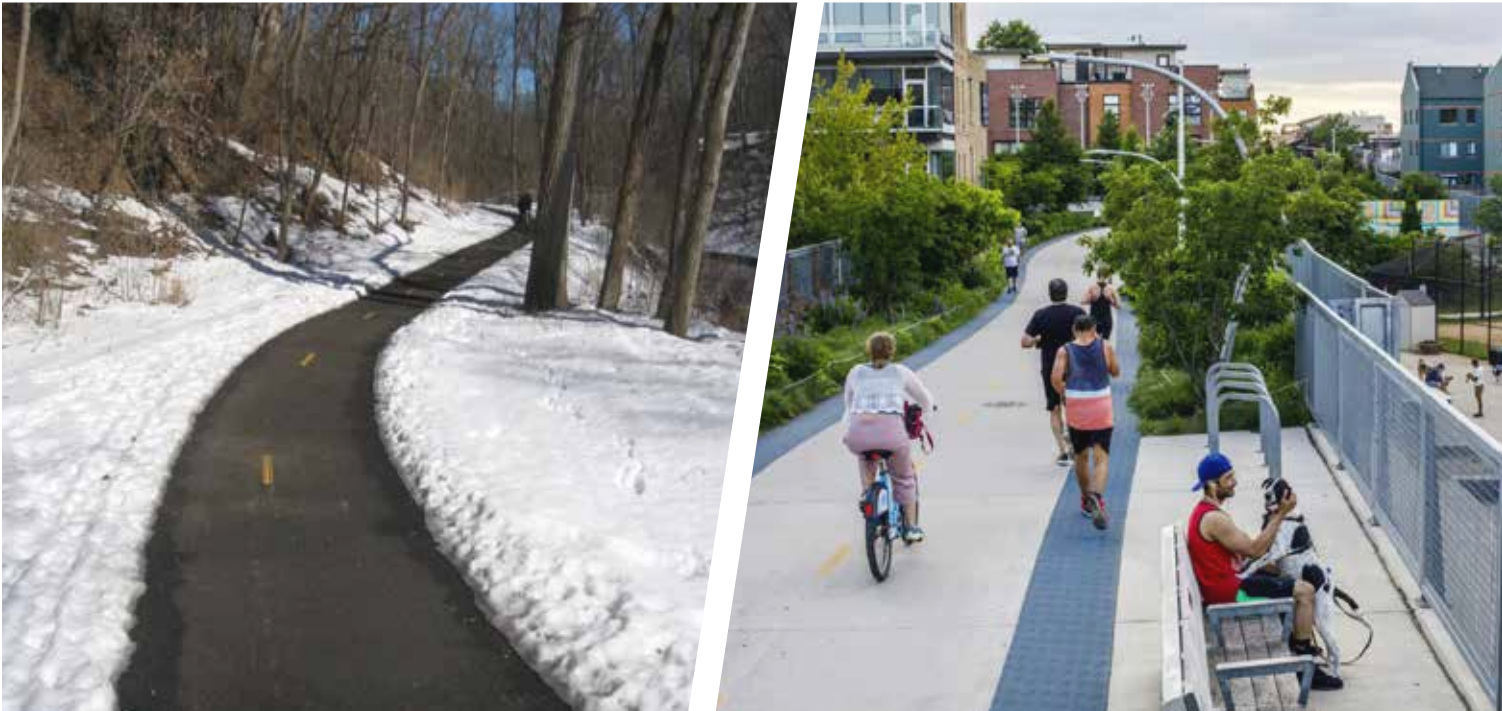
(left) Permeable asphalt, Middleton, WI; (right) Concrete with Rubber Running strip, Chicago, IL
