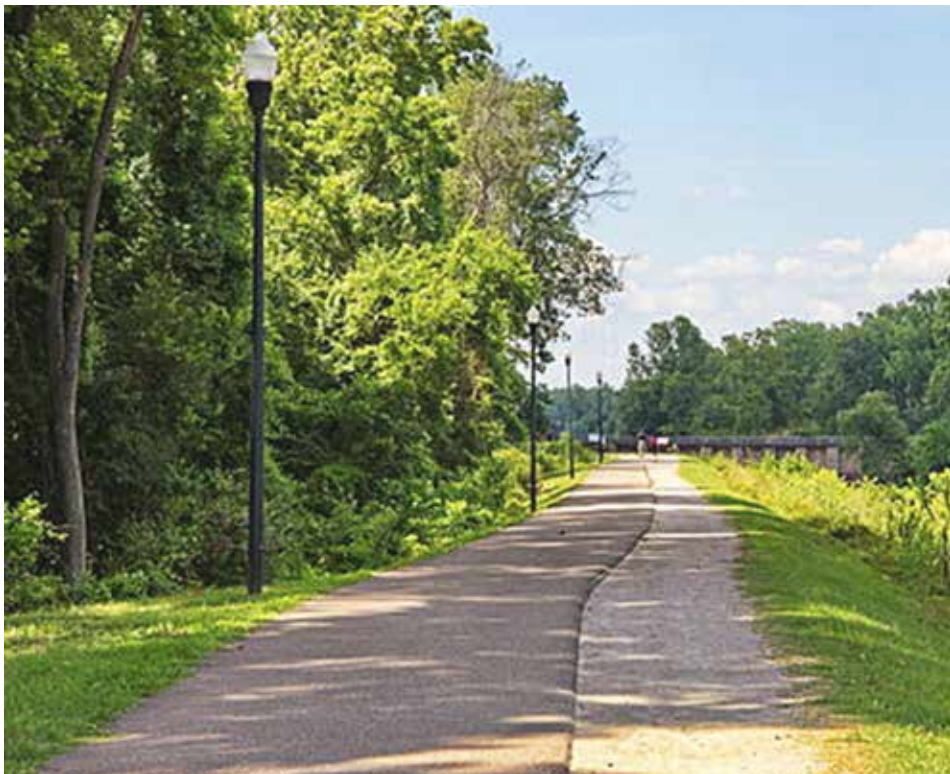
Asphalt path with aggregate shoulder, no controls
