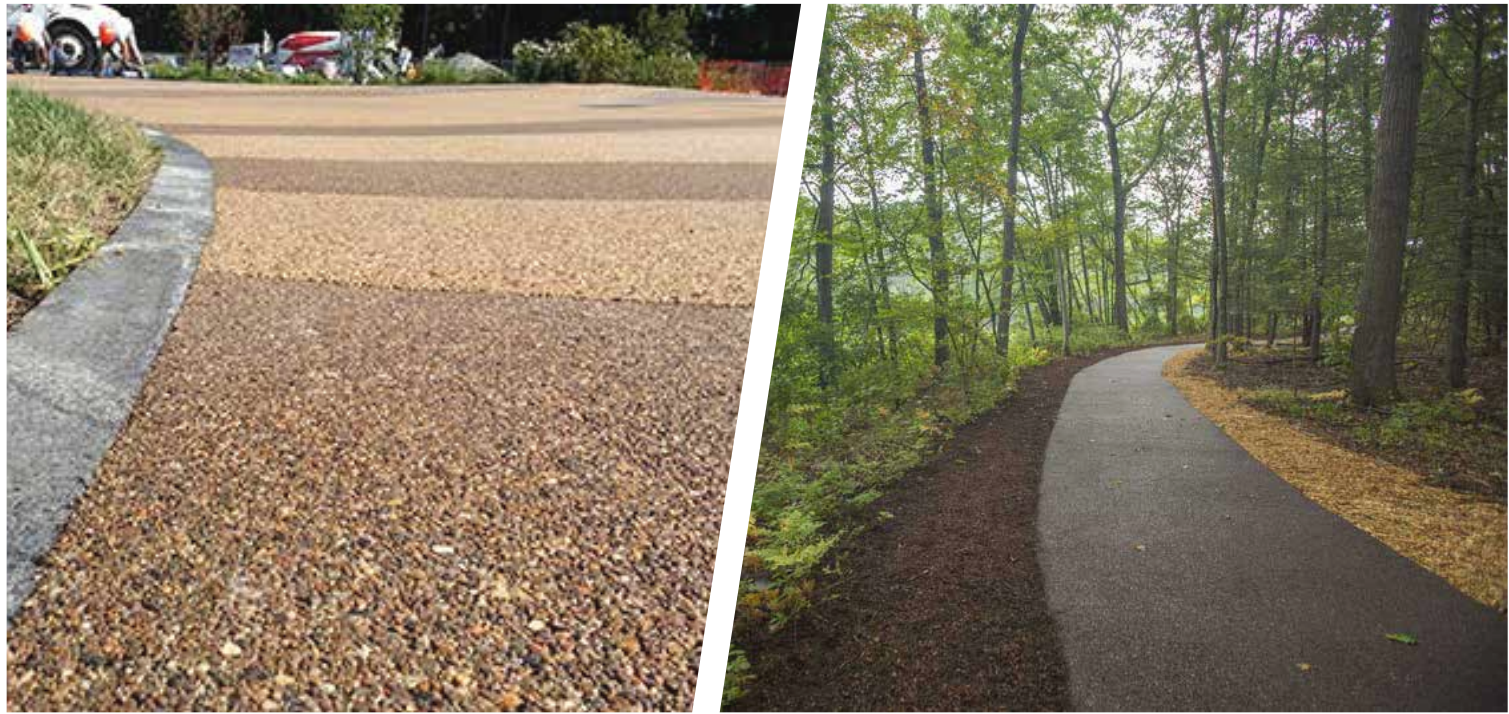
(left) Bonded Aggregate Surface Product; (right) Combined Permeable Aggregate and Rubber Surface, Wellesley, MA
