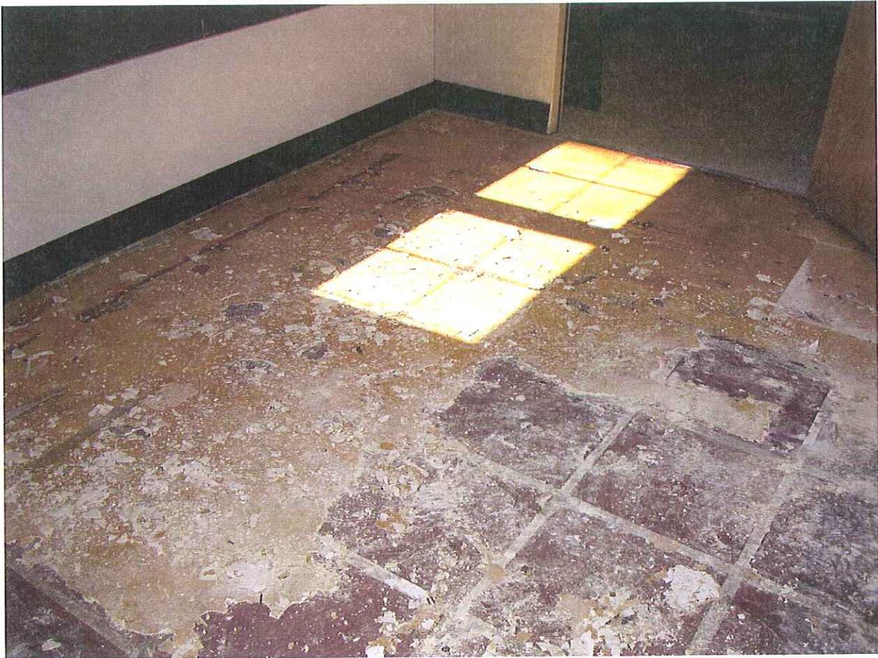
MMB 1 ST FLR. TRAFFIC ENGINEERING FLOOR
