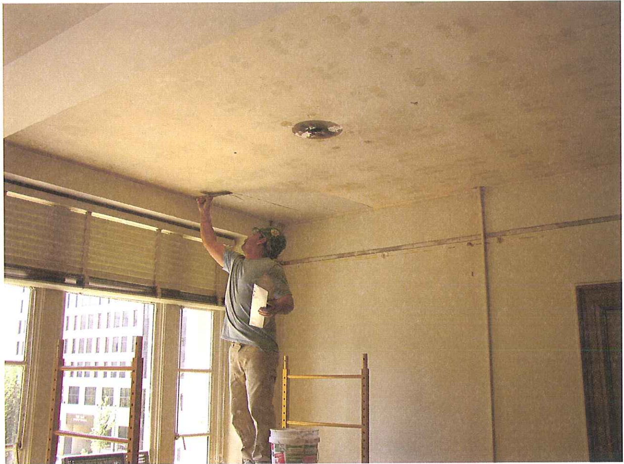
MMB 3RD FLR. CEILING SKIM COATING
