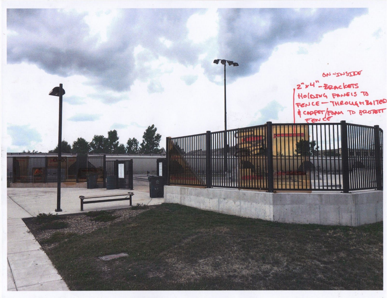
Image 5 -install option 2- wood panels attached to fence with brackets. Used painted skateboards attached to front
