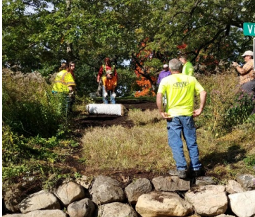
Installation of vegetated mat
