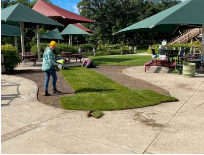
Goodman Pool Restoration
