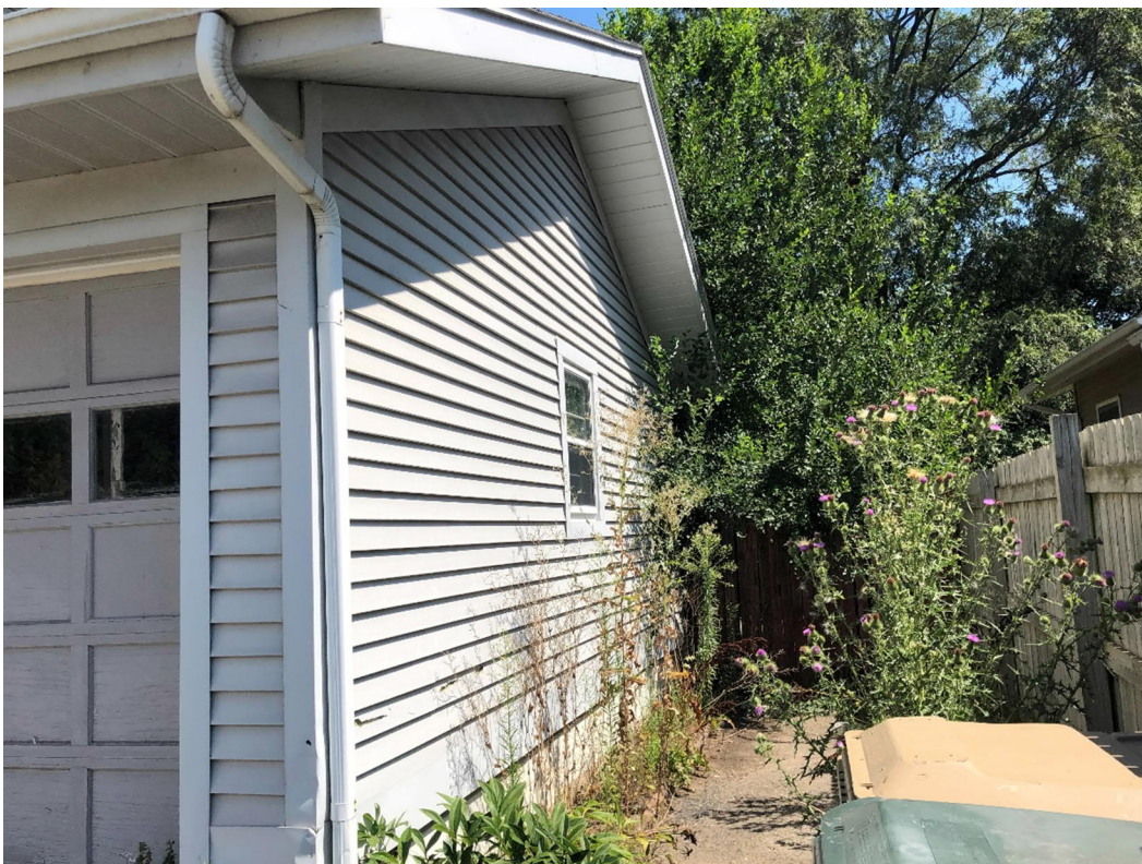
Exterior (South Side)
