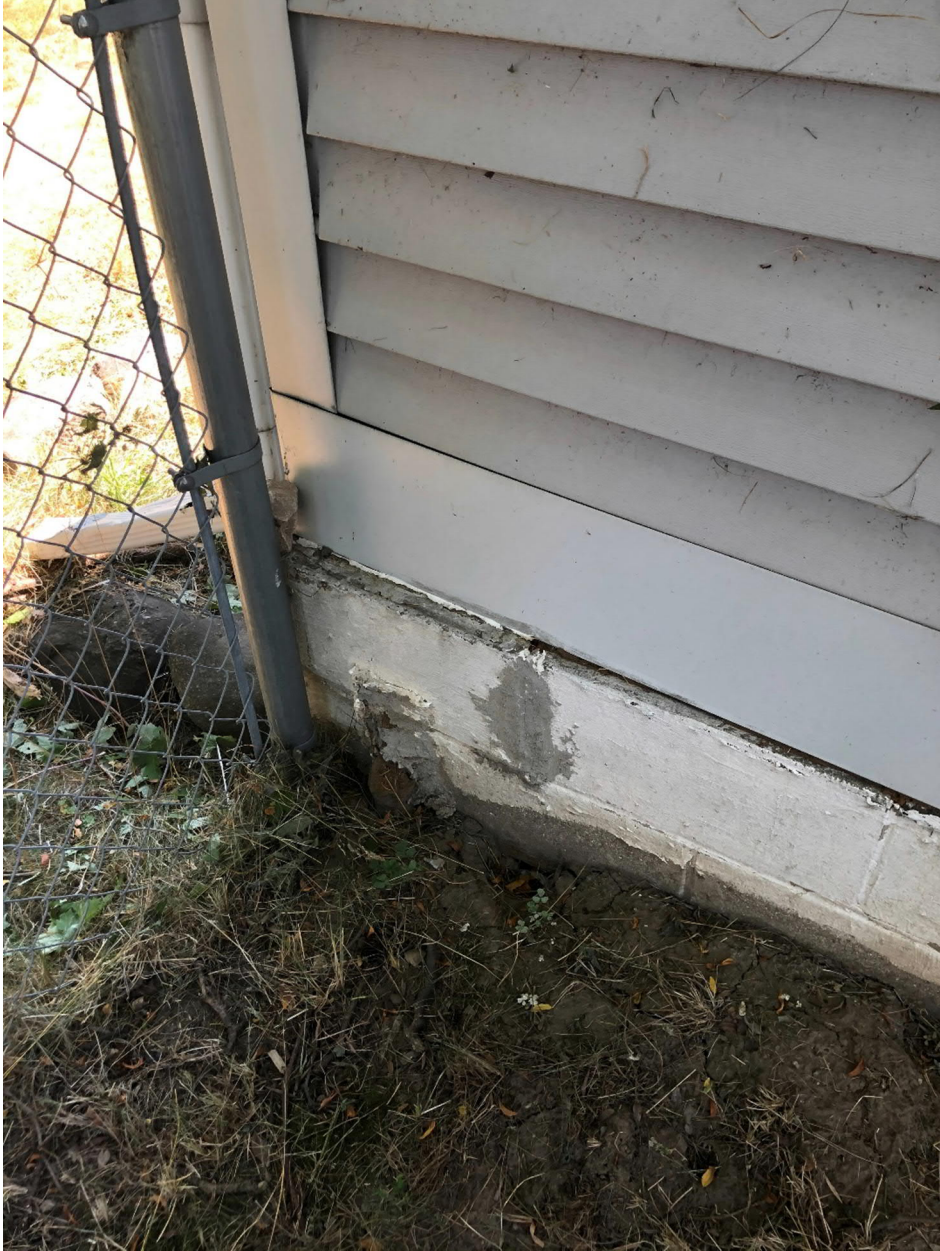
Exterior Foundation Settlement and Movement Repairs
