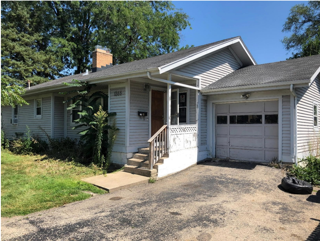
Exterior (West Side)
