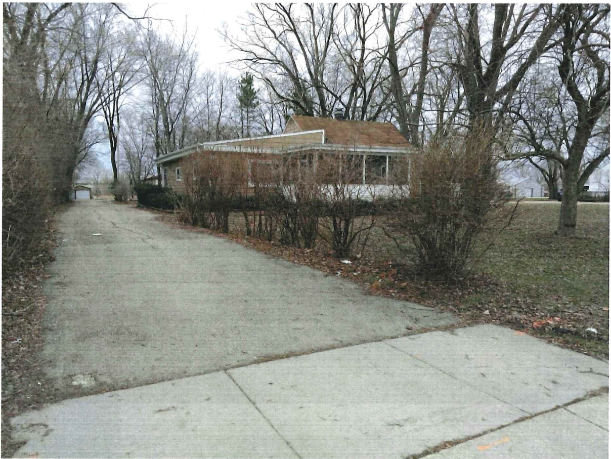
5021 at NE corner looking SW
