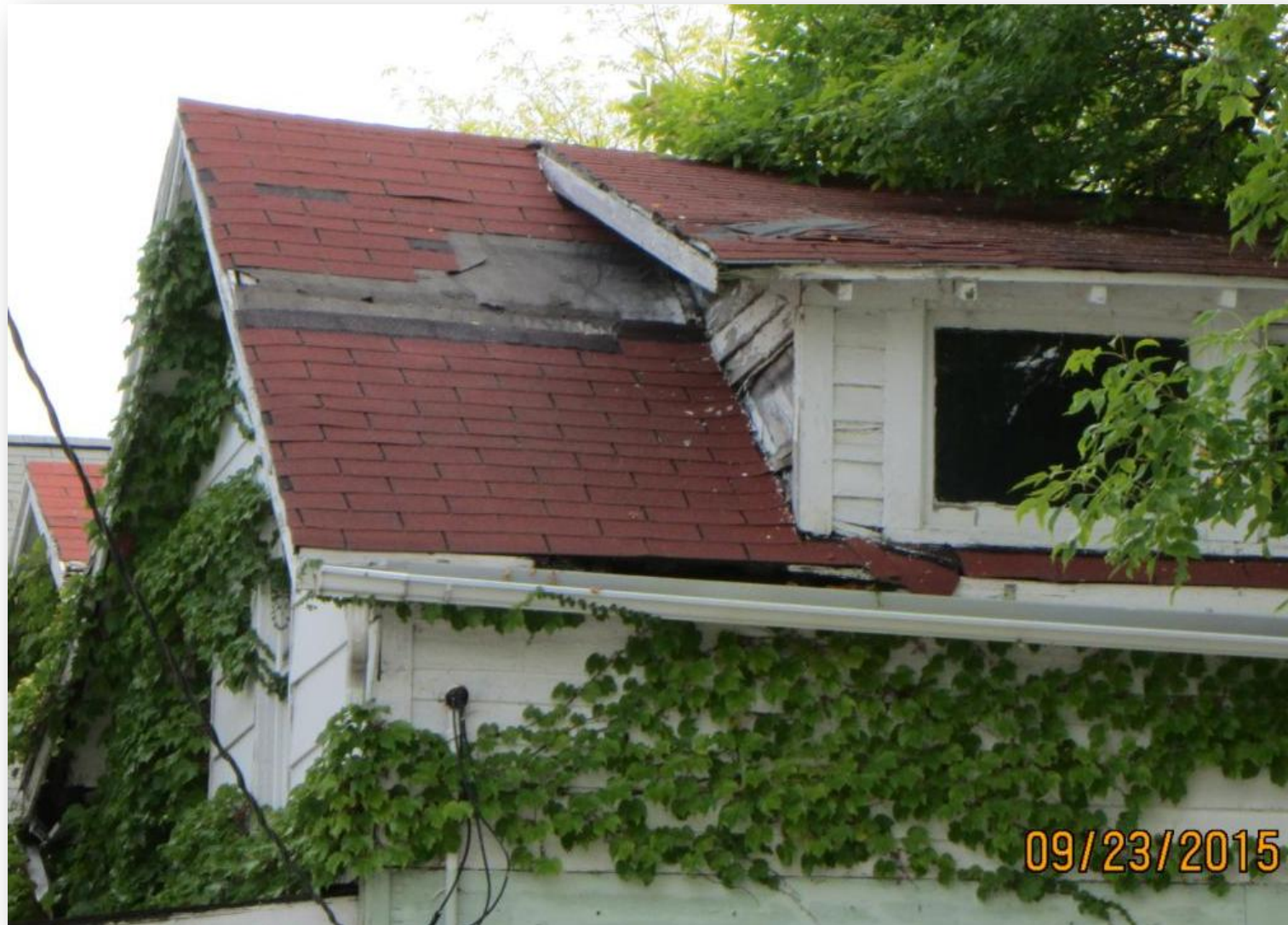
ROOF SYSTEM AND DORMER AT FRONT, WEST CORNER
