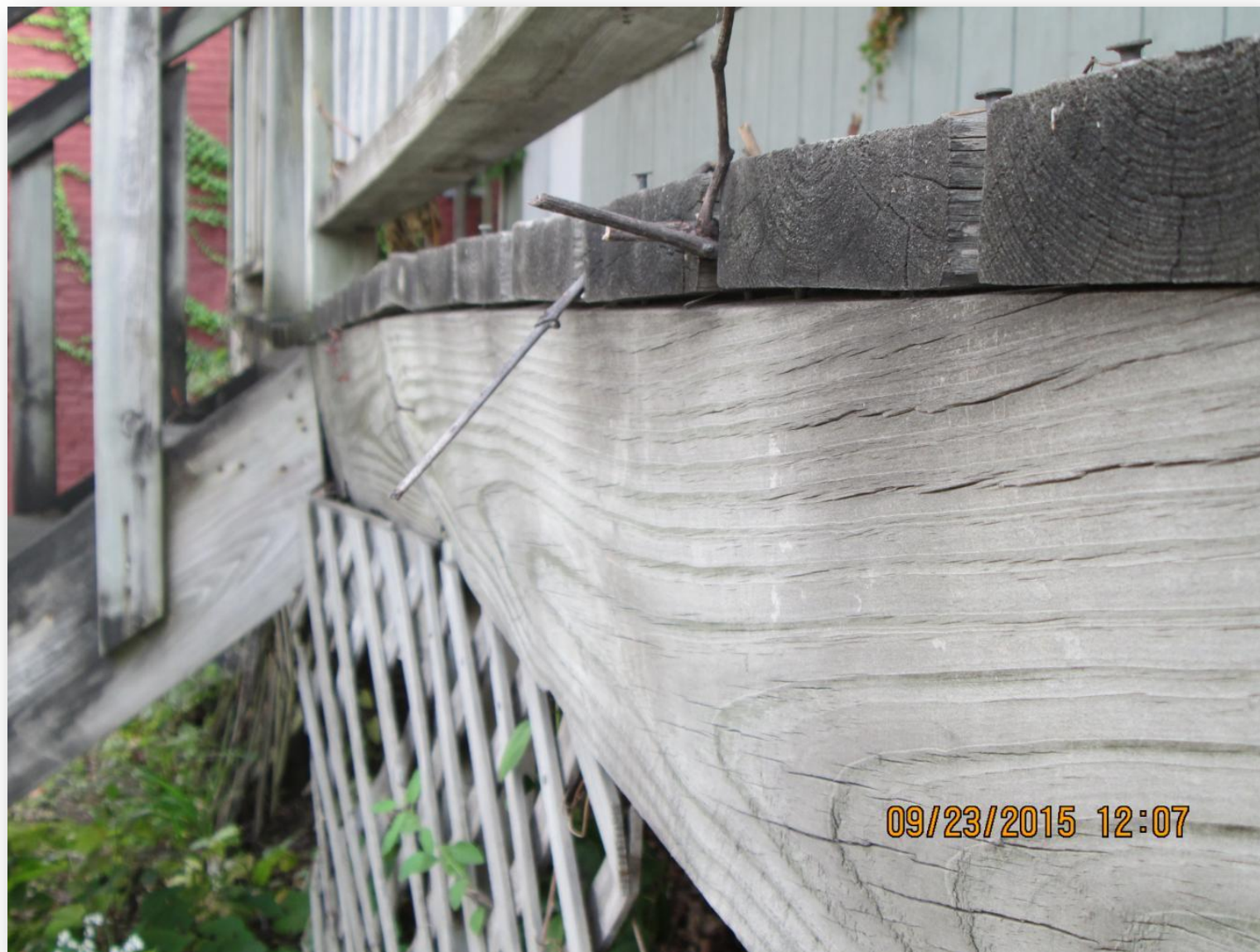
LOOKING DOWN EDGE OF FRONT PORCH FLOOR SYSTEM
