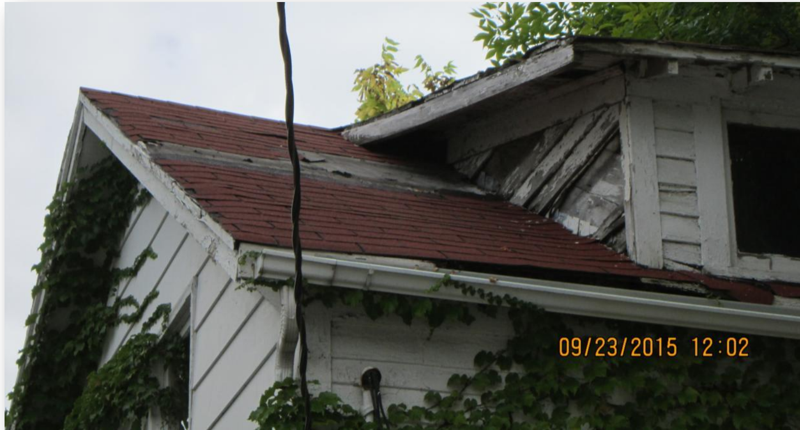
ROOF SYSTEM AND DORMER AT FRONT, WEST CORNER (2)
