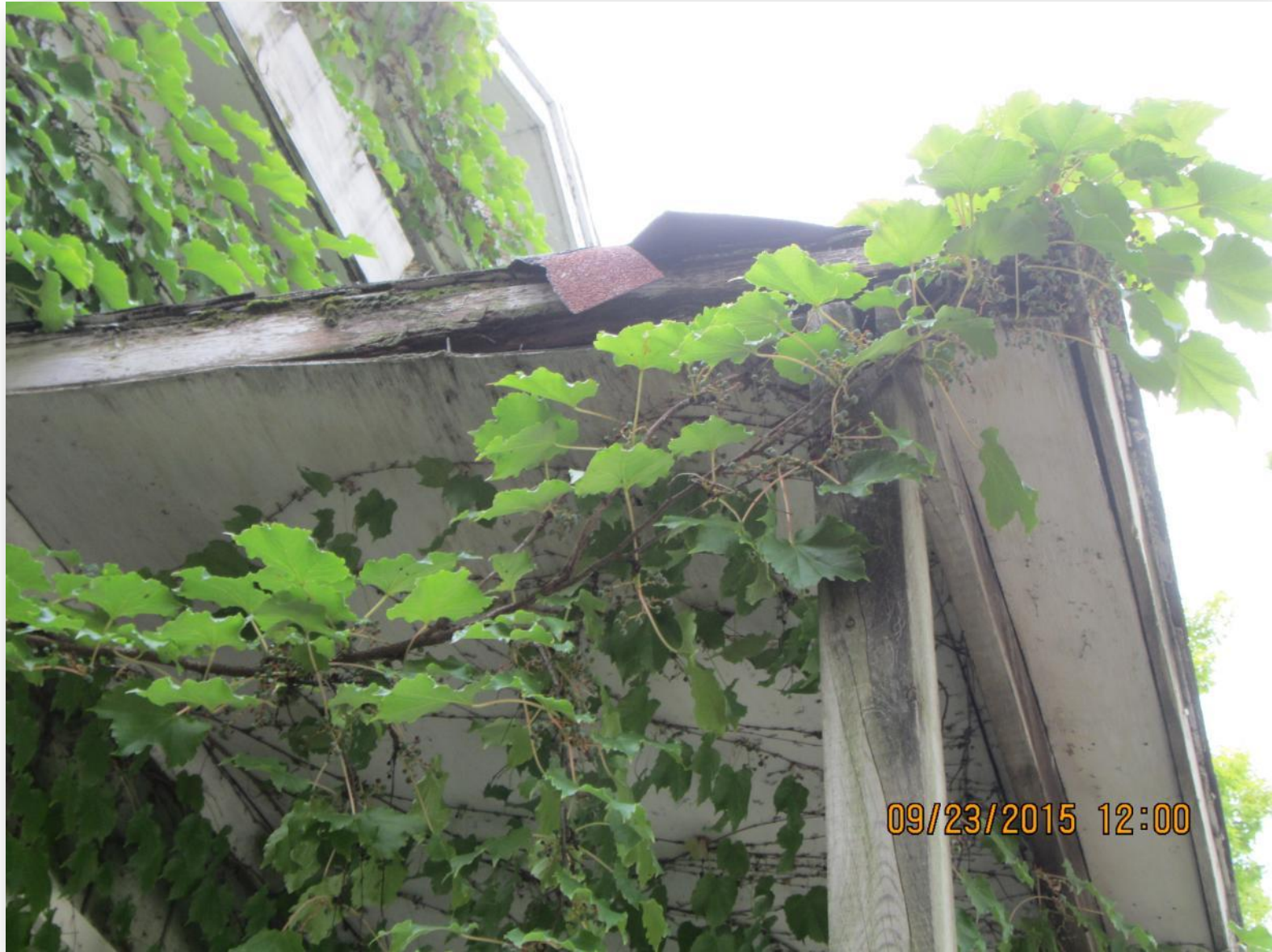
EAST SIDE OF FRONT PORCH ROOF
