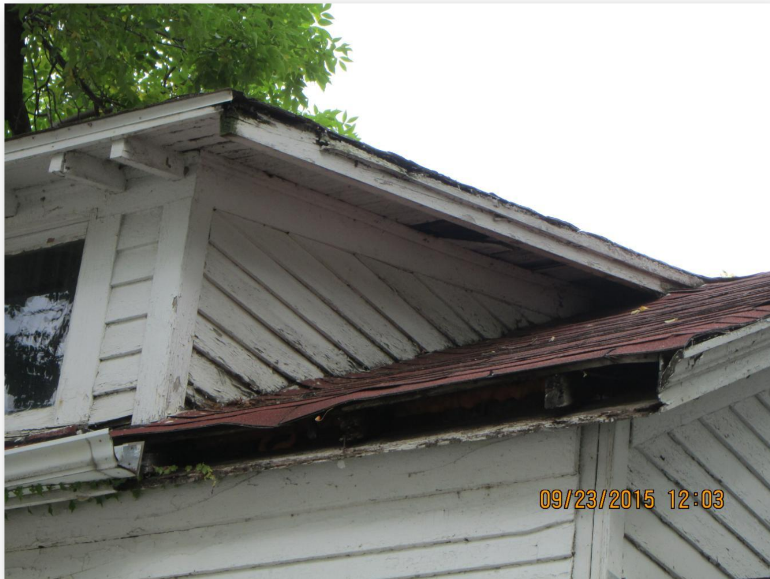
ROOF SYSTEM AND DORMER AT WEST, REAR CORNER (2)
