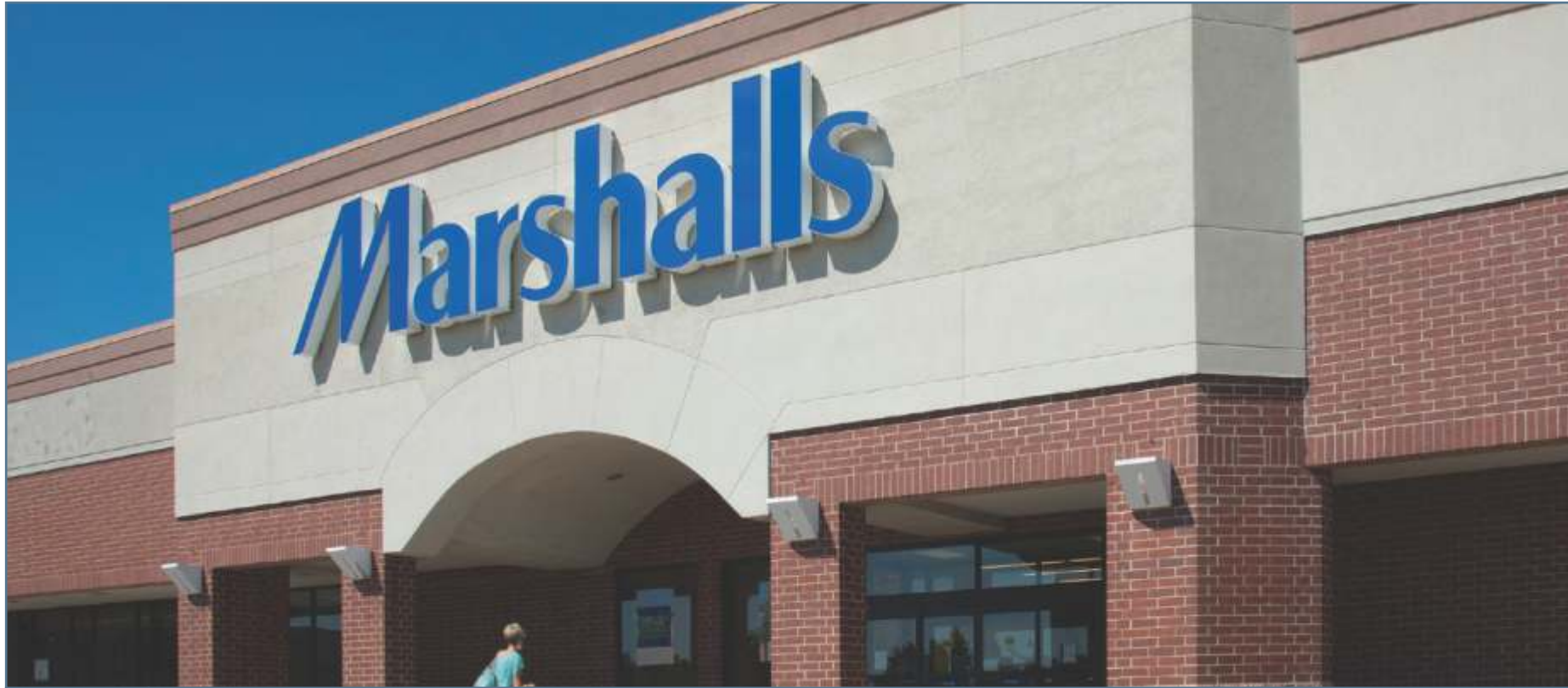
EXHIBIT 9 MAJOR TENANT WITHIN EAST TOWN PLAZA (MARSHALLS)
