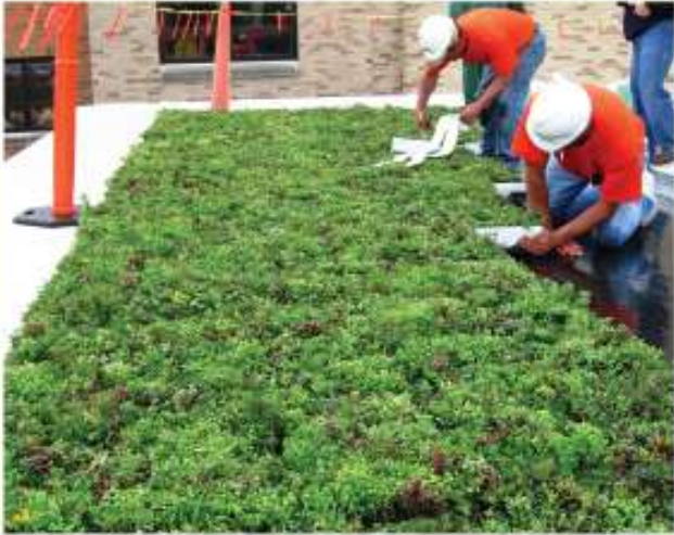
LiveRoof® modules eliminate air gaps and are protected from harmful UV rays to prevent photodegradation.
