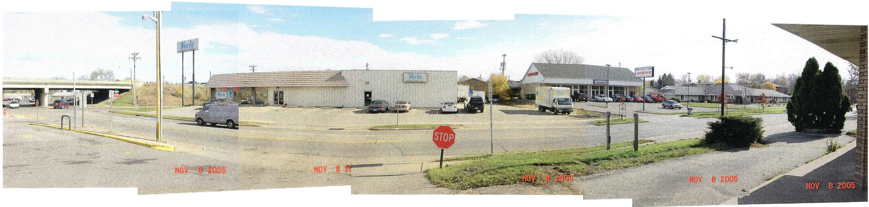
neighboring buildings to the east
