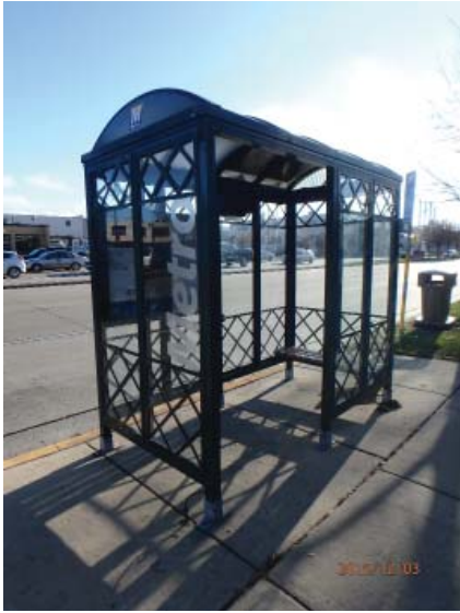
Bus Stop at East Washington and North Ingersoll (paint chipping, graffiti)
