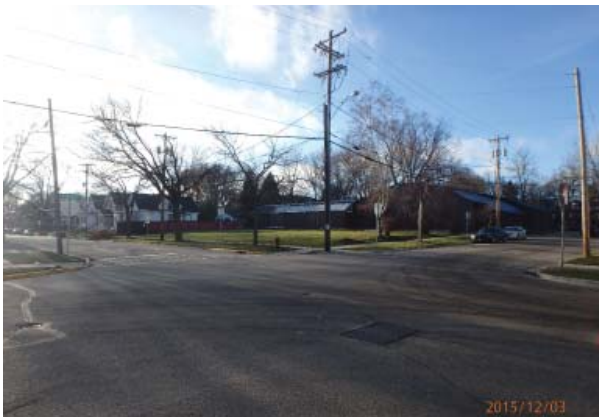
North Dickinson at East Mifflin looking southeast (cracking, patching, paint chipping)
