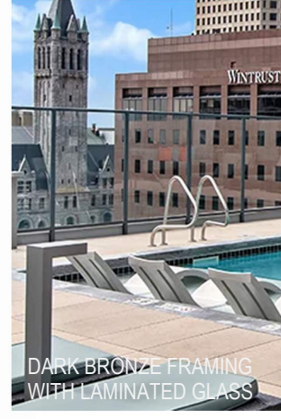
GLASS GUARDRAIL ASSEMBLY
