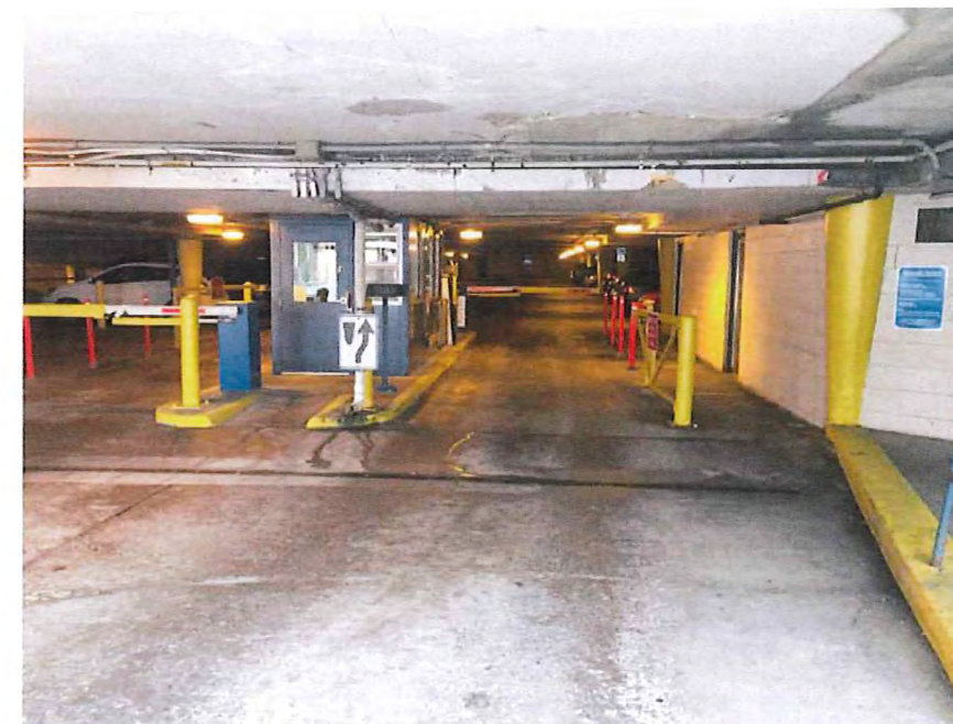
Existing Interior at Wilson Street Entrance
