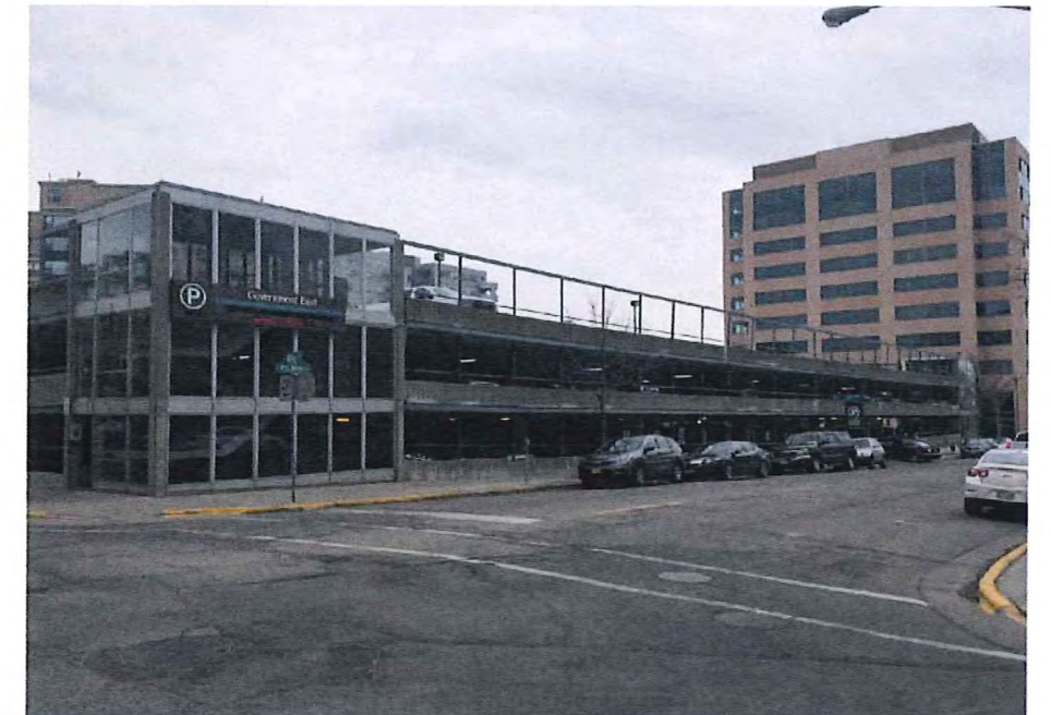
Existing Exterior Along Pinckney Street
