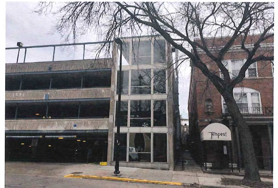
Existing Exterior at East End of Wilson Street
