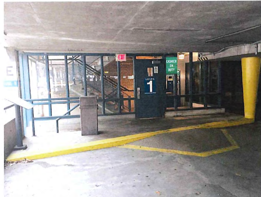
Existing Interior at North Corner of Garage
