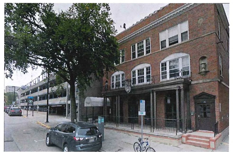
V7 - Existing site from E Wilson Street
