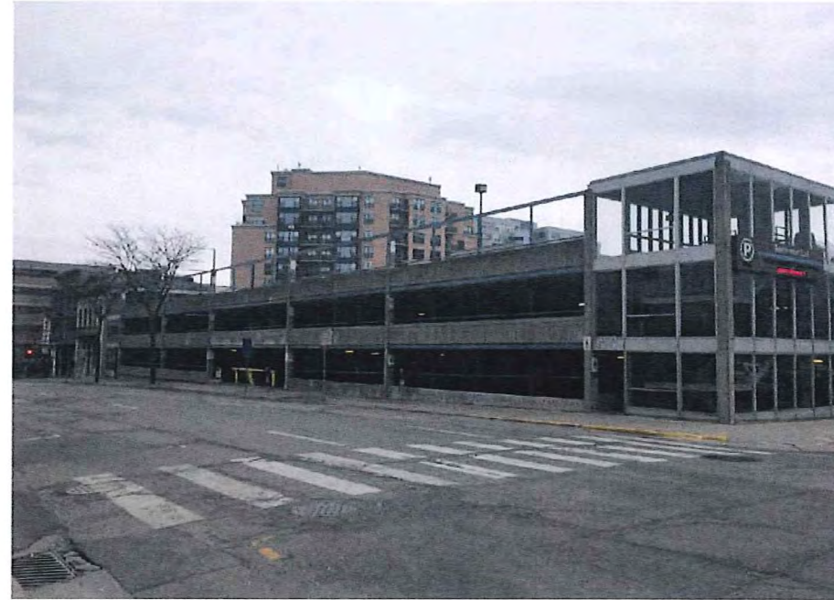
Existing Exterior Along Doty Street
