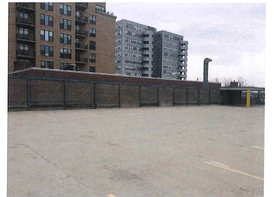
Existing Interior at Rooftop Looking East
