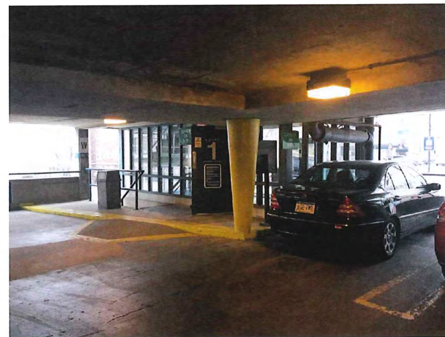
Existing Interior at South Corner of Garage
