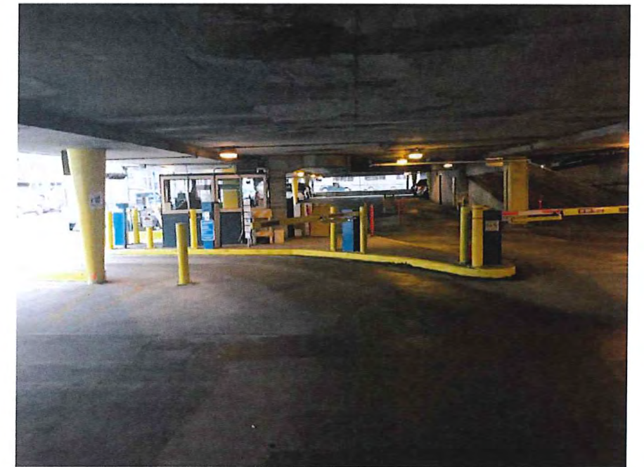
Existing Interior at Pinckney Entrance
