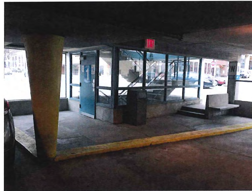
Existing Interior at West Corner of Garage
