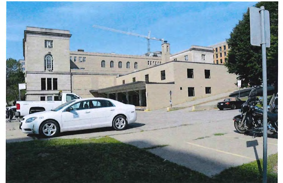
V6 - Existing site & MMB from Pinckney Street
