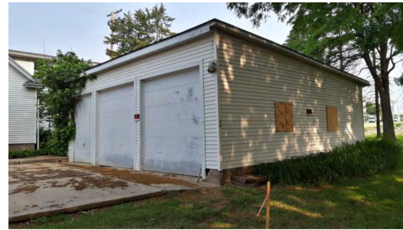
VIEW OF GARAGE LOOKING NORTHWEST.
