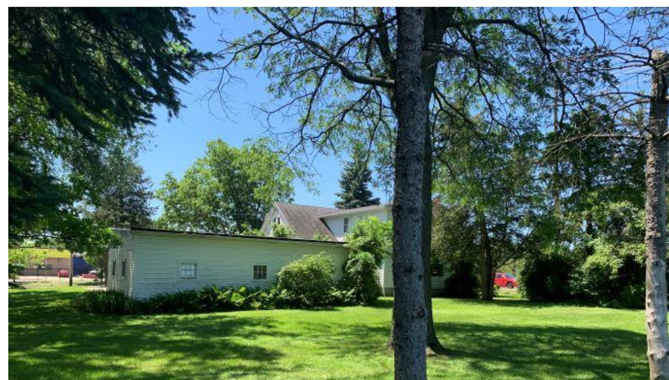
VIEW OF GARAGE AND HOUSE LOOKING SOUTHWEST.
