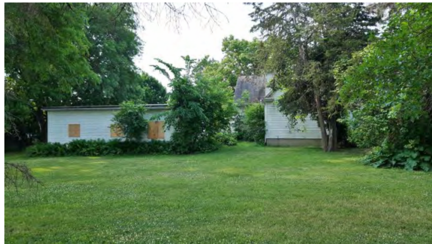
VIEW OF GARAGE AND HOUSE LOOKING SOUTH.
